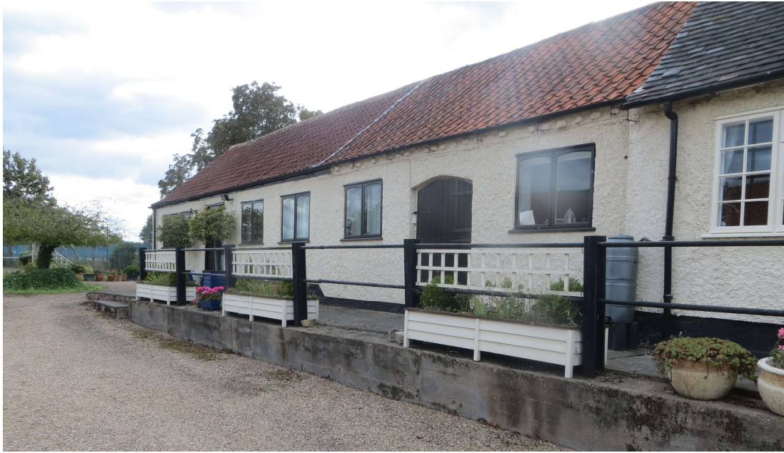
Figure 4 – Rectory Farm, east elevation to yard
