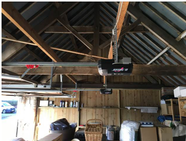
Garage interior looking north
