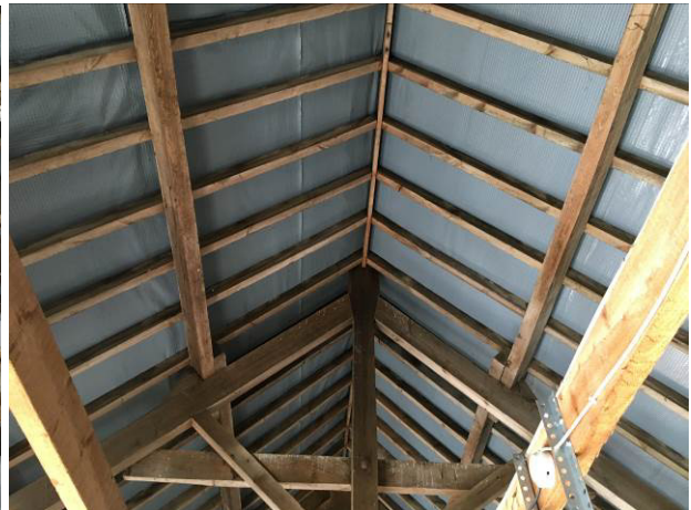
Interior of garage roof
