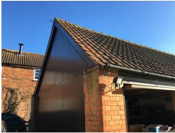
North gable and roof
