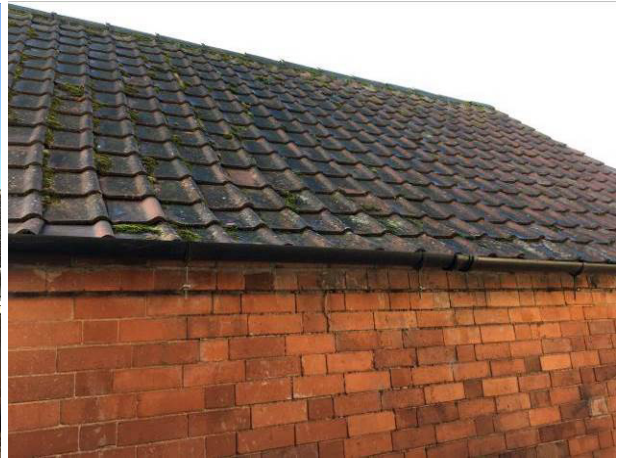
Roof to rear of garage
