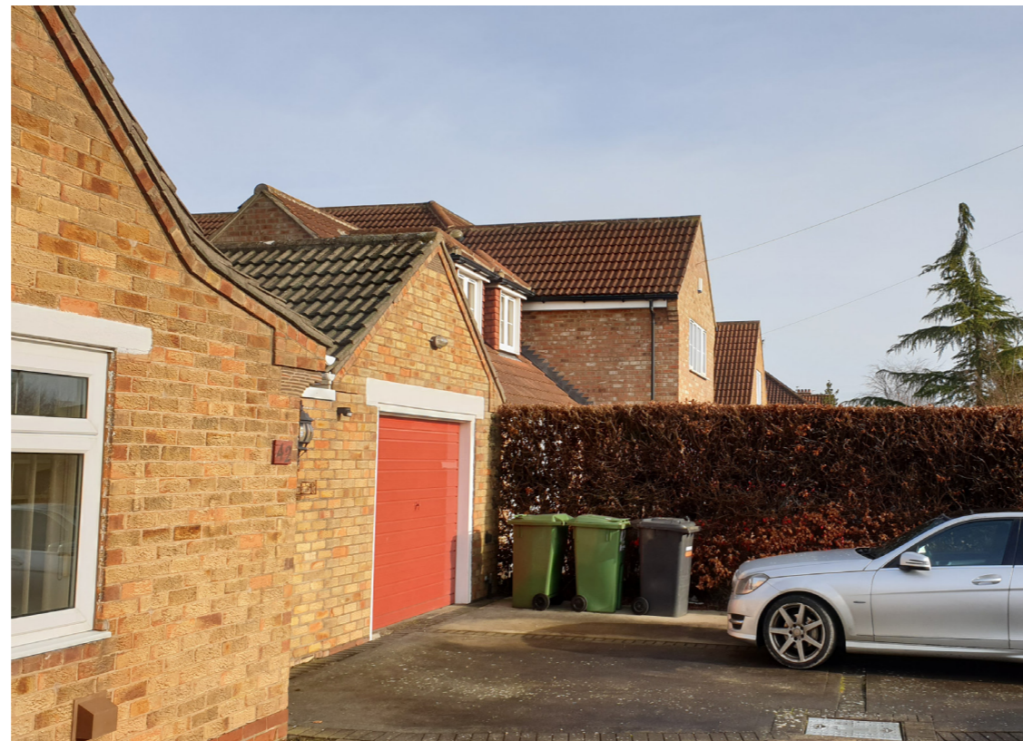
image b - part 1, part 2 storey home adjacent
