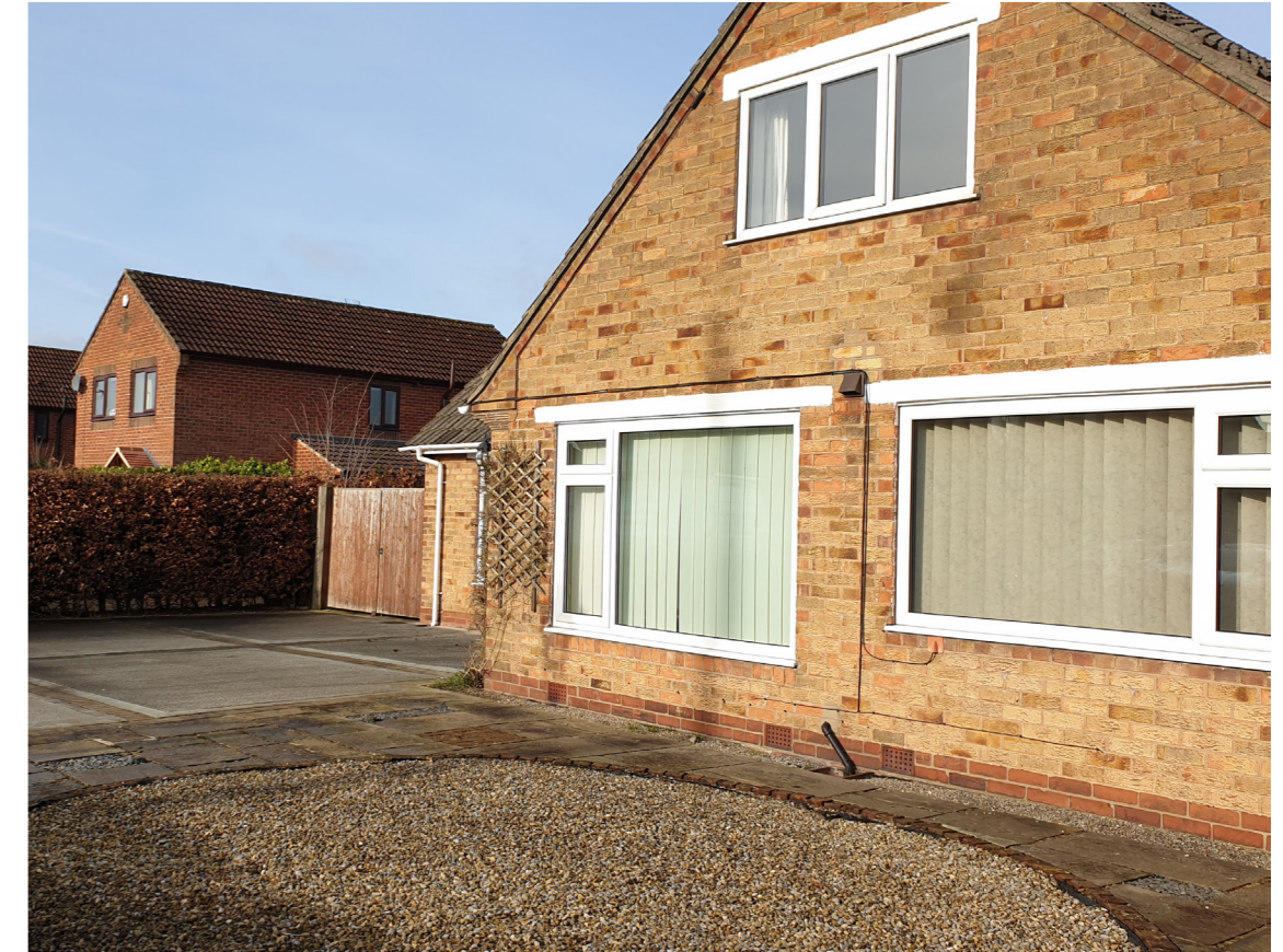
image a - 2 storey home adjacent
