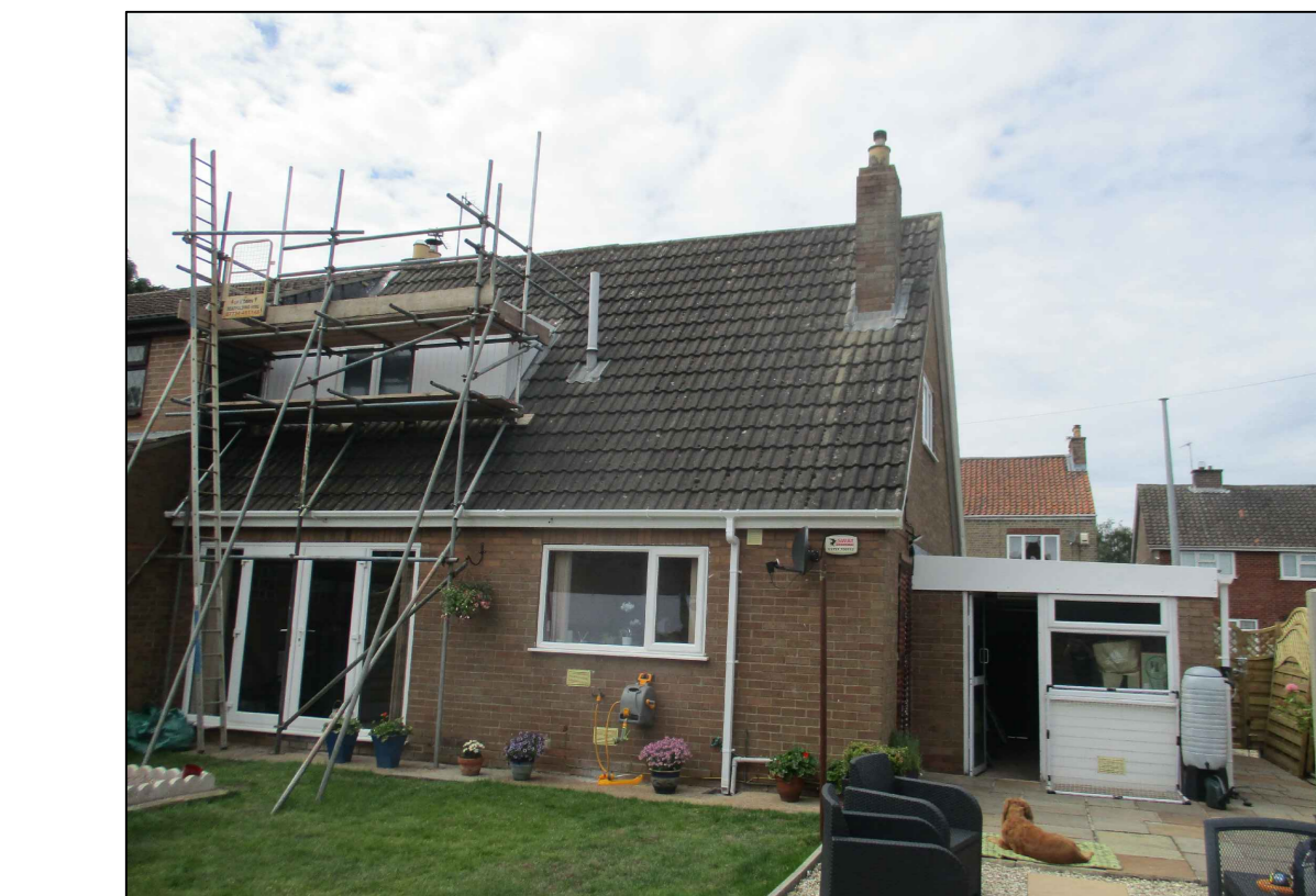
EXISTING REAR IMAGE 03
