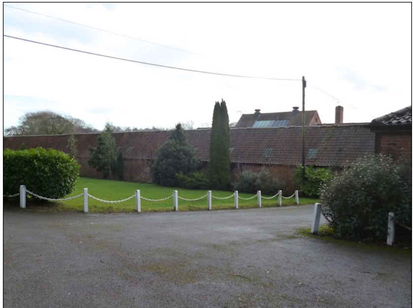
Photo 8: View of the rear wall of the northern range of The Courtyard buildings from Lound Hall with the roof of the southern range in the background
