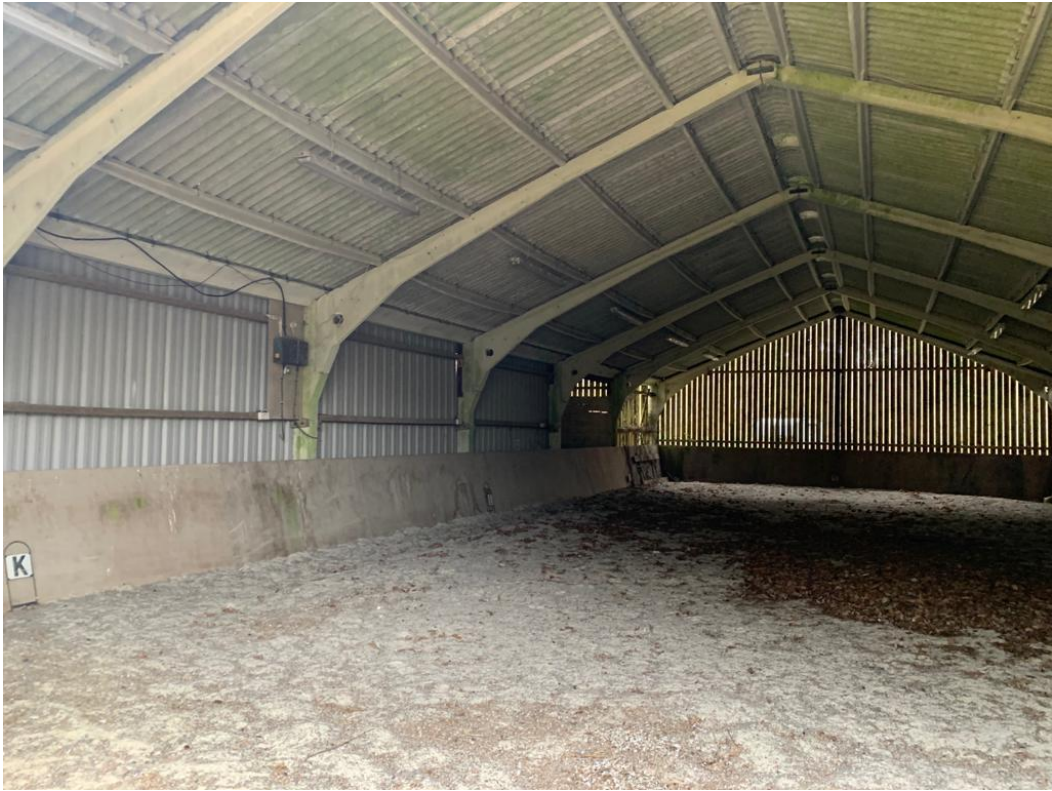
Further view inside horse exercise building (building 1)
