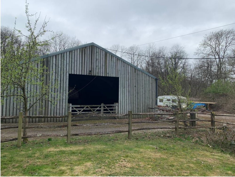
View of horse exercise building (building 1)
