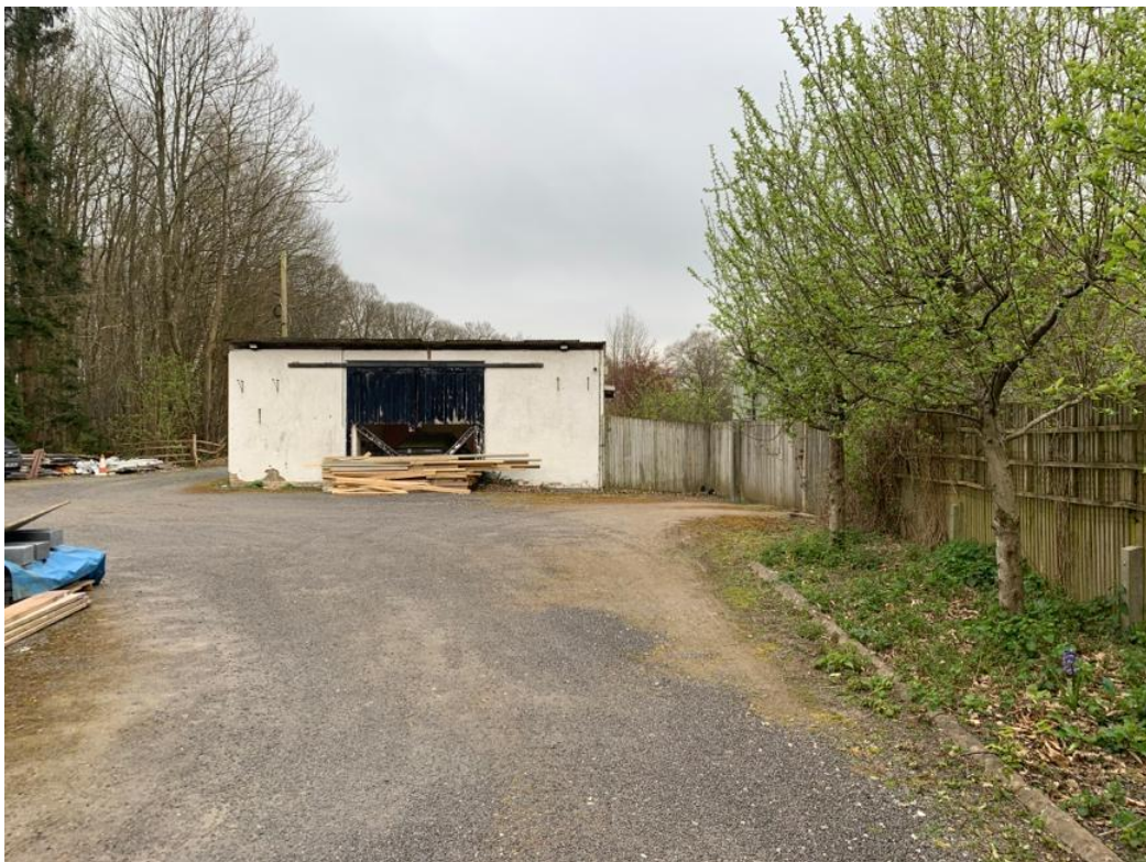
View from access towards building 4
