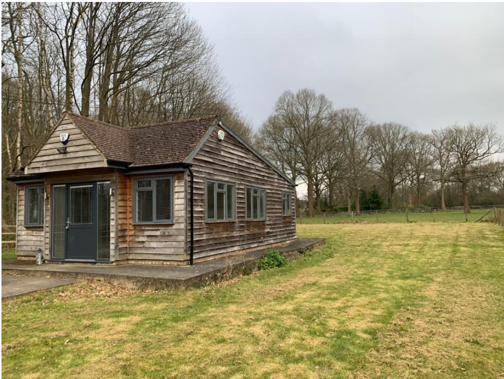
View of office building (building 3)
