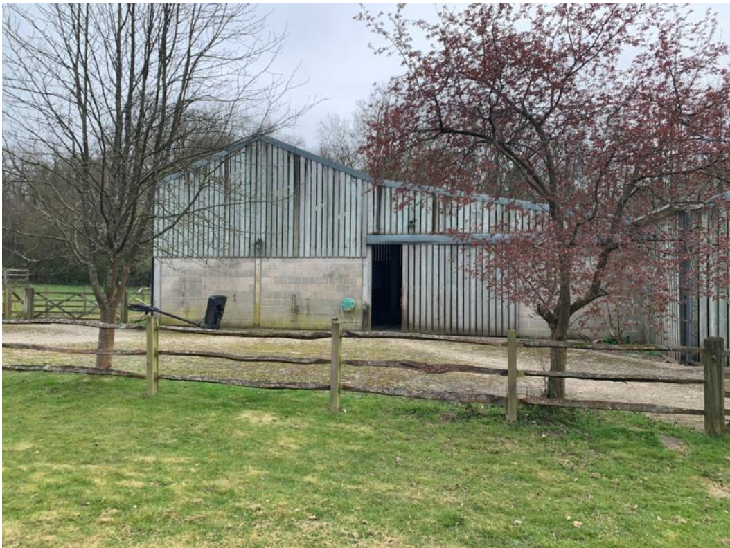
View towards building 2 (the stable building)
