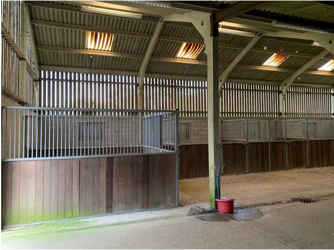
View inside stable building (building 2)
