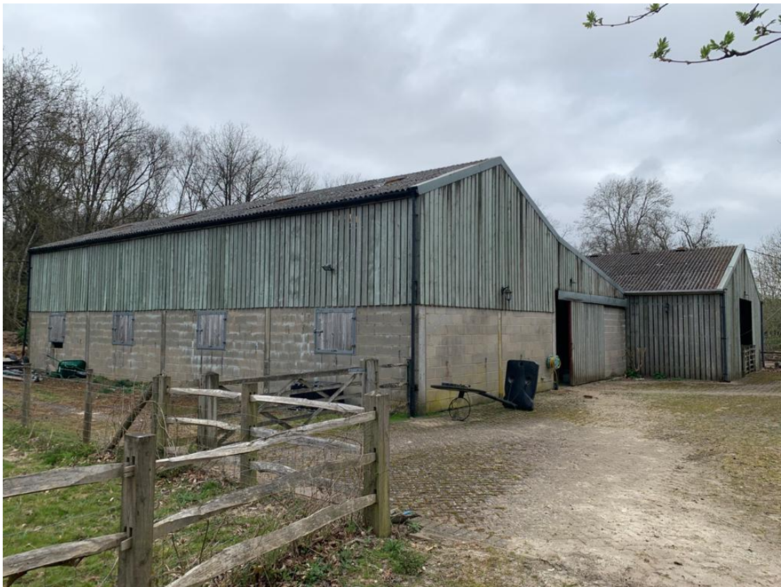
View towards buildings 2 (foreground) and building 1 (background)
