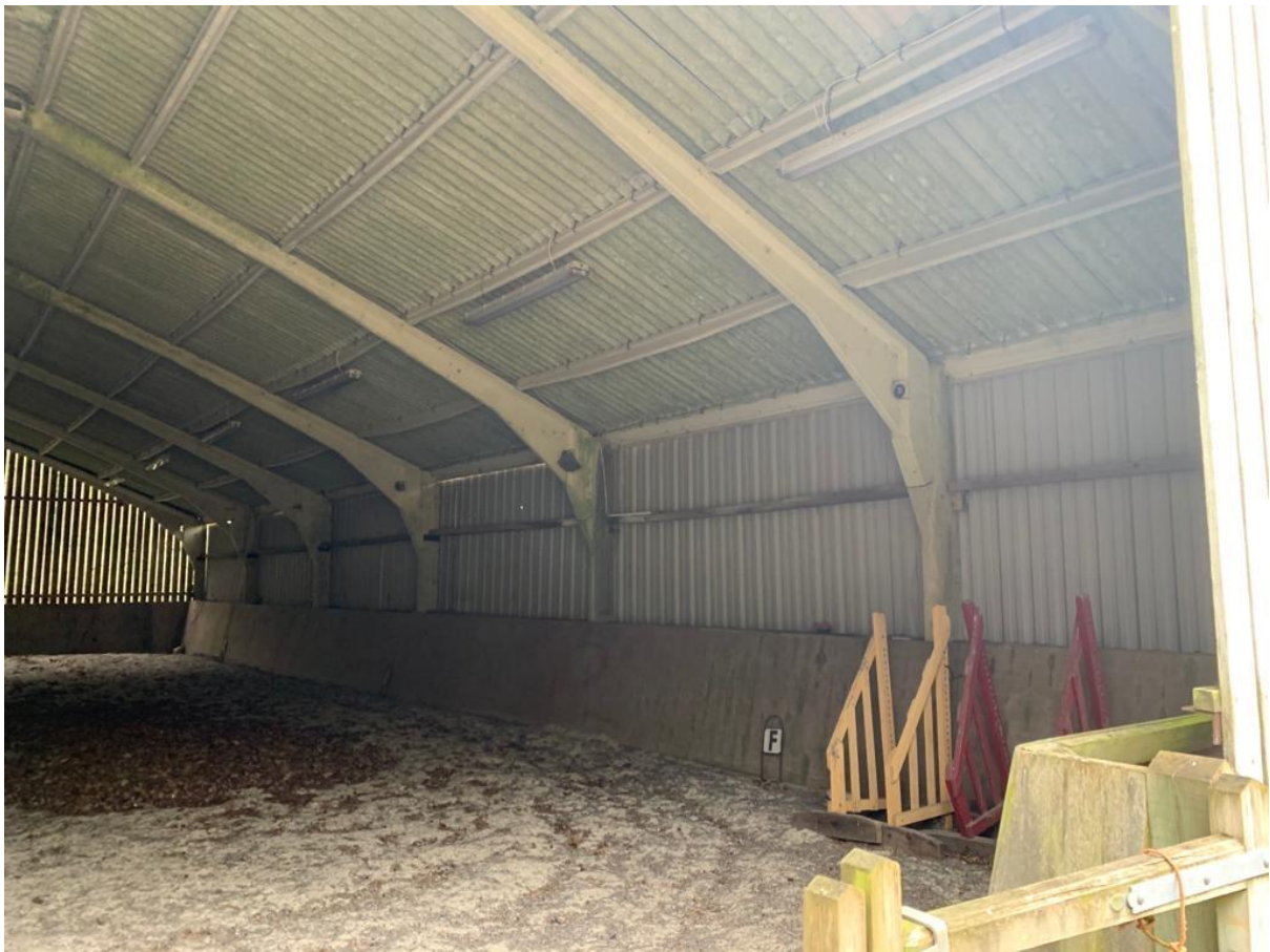
View inside horse exercise building (building 1)
