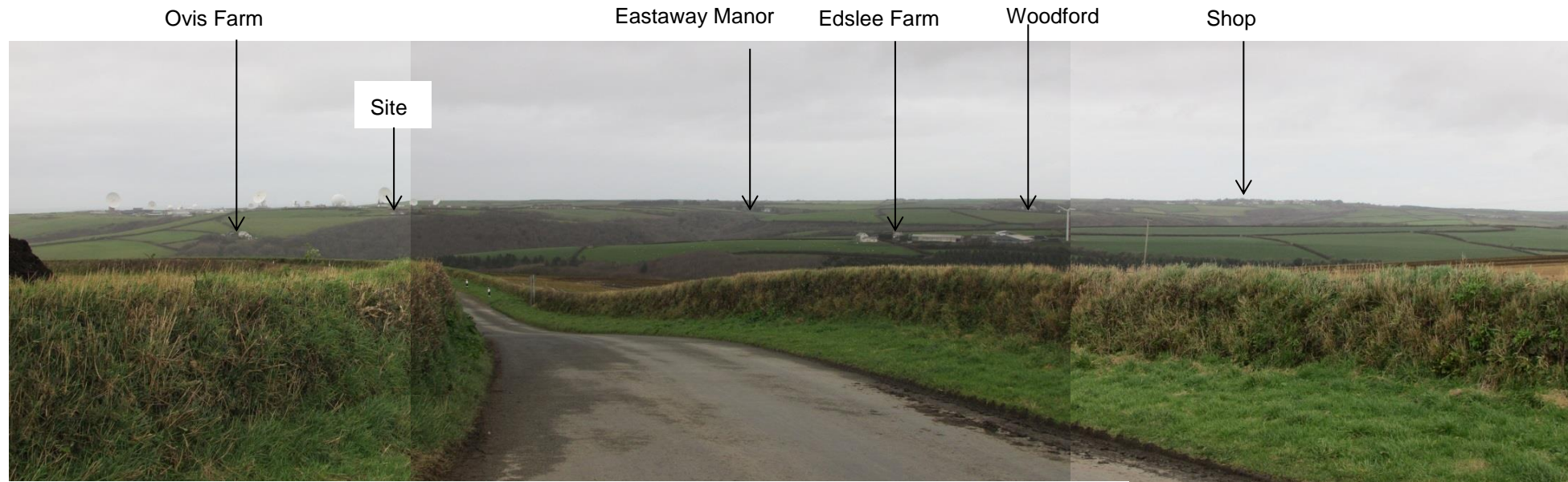
VIEW X - (VP 21) Looking north on Stibbs to Coombe Road near Junction to Houndapitt Farm along access track to site
