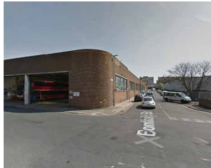
Brighton & Hove Bus workshop, East Garage, Conway Street Image Source: Google
