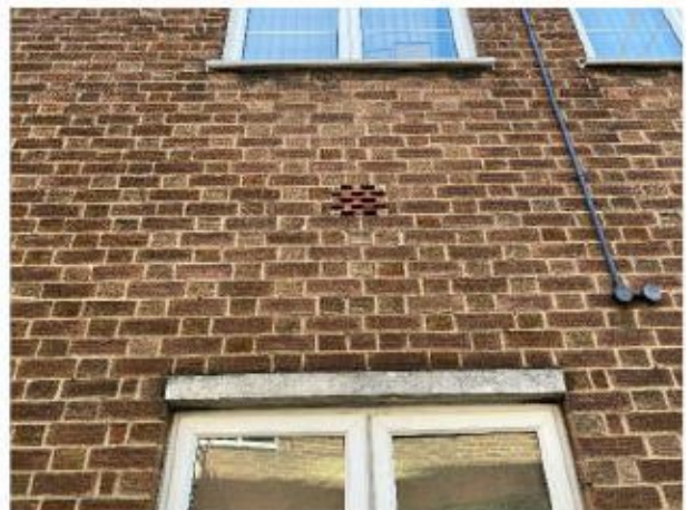
Ventilation holes built into external walls
