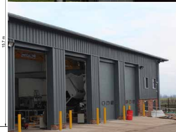
Examples of panelling facade
