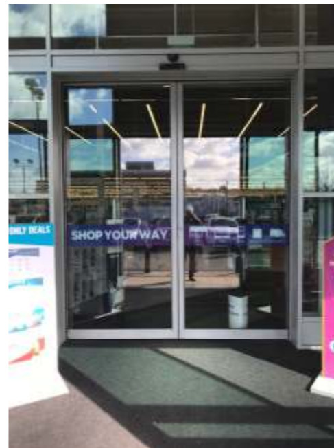
6 LOBBY - ENTRANCE EXISTING
