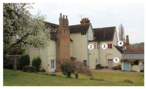
Elevations showing windows to be replaced. Numbers relates to window/door types as shown on WM(3-)01 Windows Replacement Proposal drawing.
