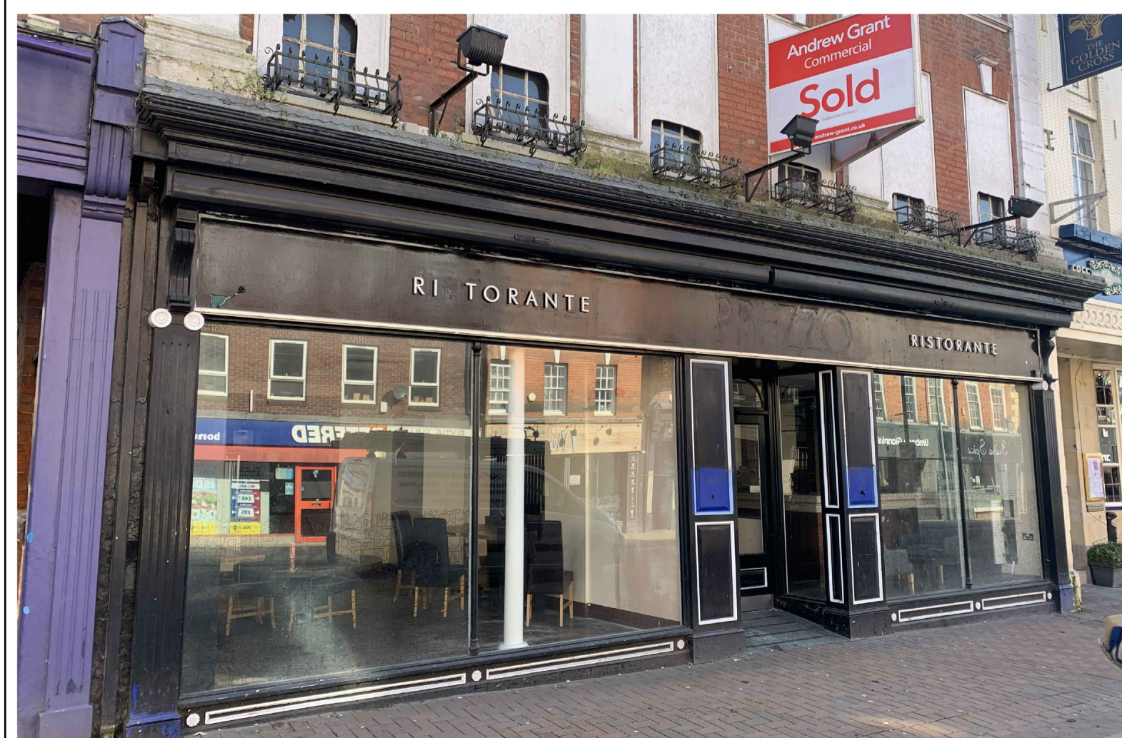
EXISTING ELEVATION PHOTOGRAPH
