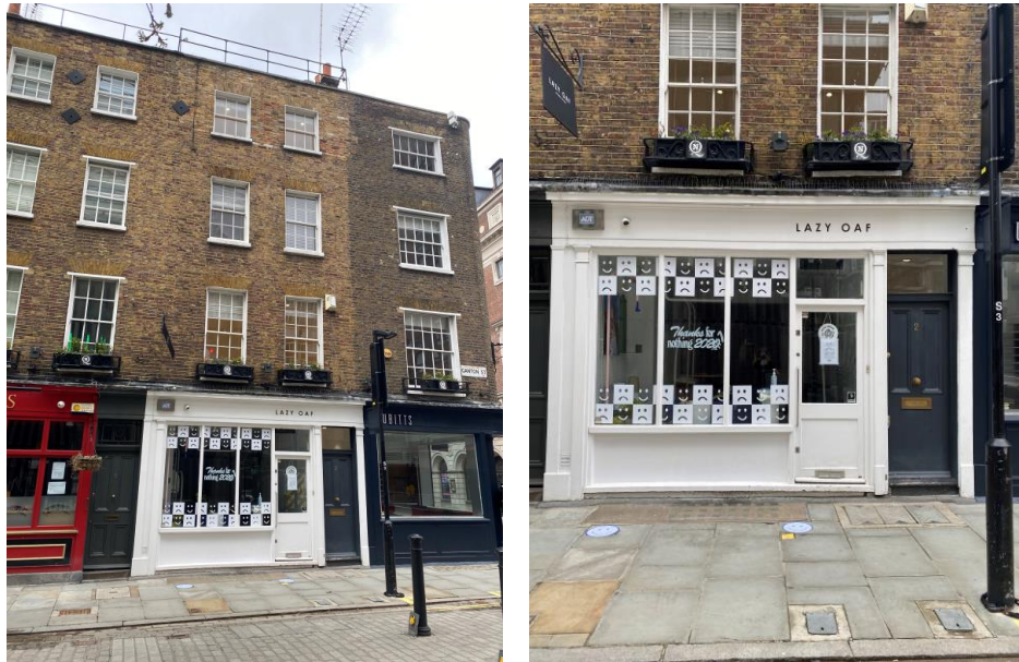
Figures 8 and 9: Front elevation and shopfront of 2 Ganton Street
