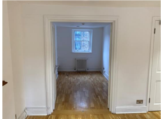
Figures 14 and 15: Third floor at 2 Ganton Street showing the modern fire surround (left) and opening in the spine wall (right)
