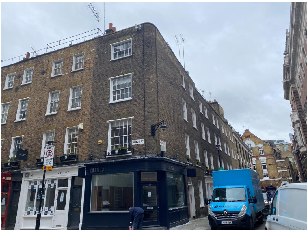
Figure 1: 37 Marshall Street (grade II)
