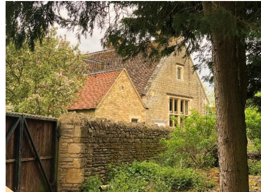
View of rear upon approach from Church. Note the flat roof is fully concealed from sight.
