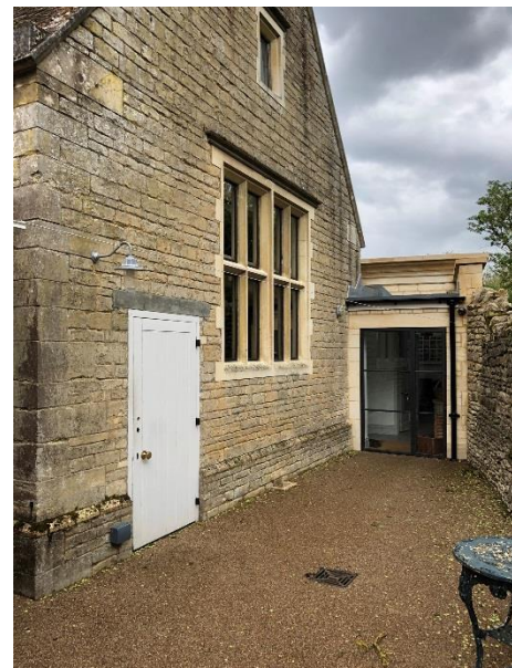
Rear courtyard view towards 2019 kitchen extension
