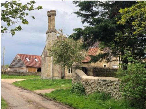
View of rear upon approach from Church. Note the flat roof is fully concealed from sight.
