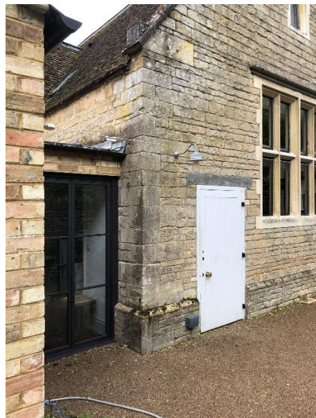
Rear courtyard view of concealed flat roof area
