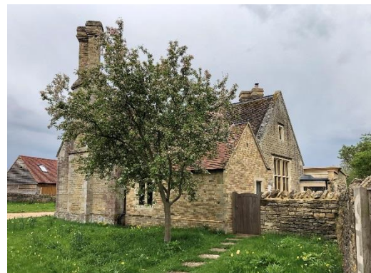
View of rear upon approach from Church. Note the new Roof Window is fully concealed from sight.
