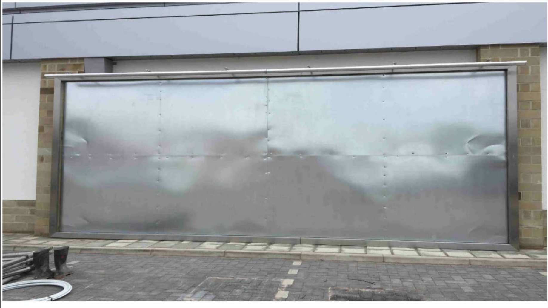
Daylight View of Typical Billboard Frame
