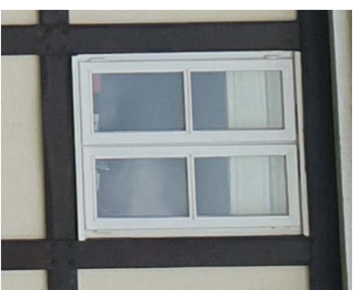
EXISTING WHITE TIMBER FRAME WINDOWS
