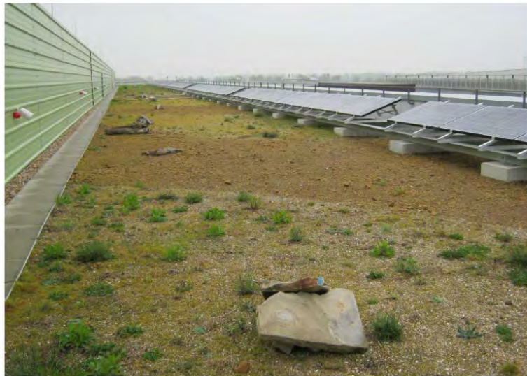
Figure 3 Green roof at the Queen Elizabeth Olympic Park (University of East London)
