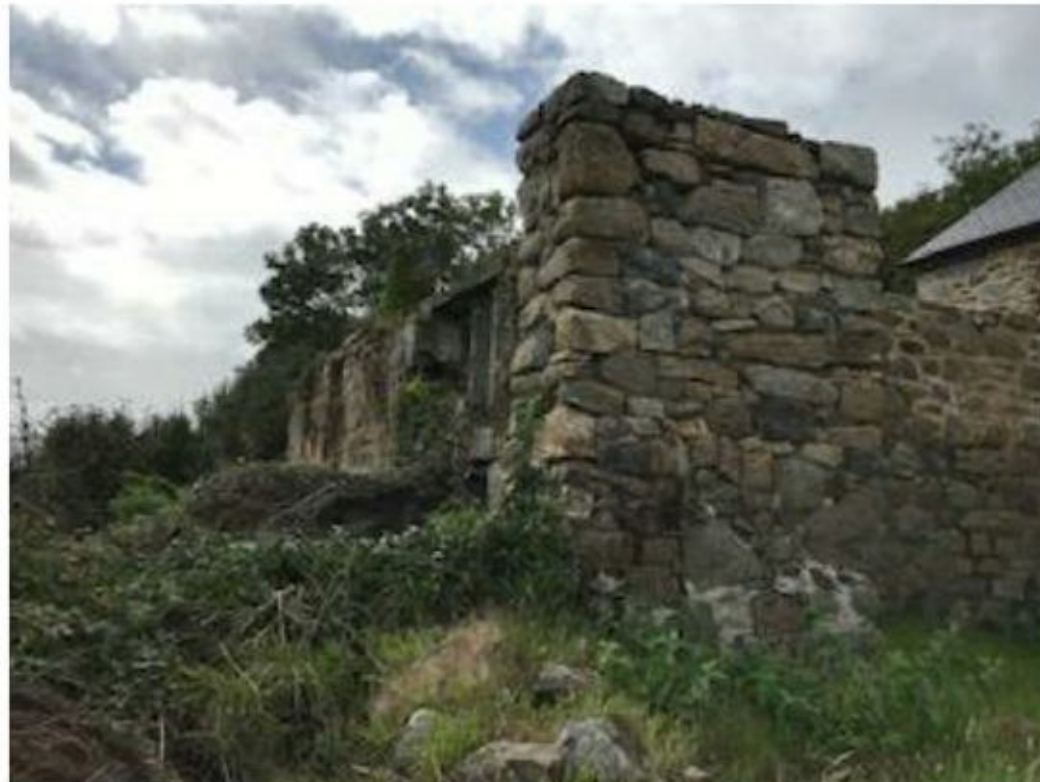
Photo 1: South-eastern corner of the cottage
