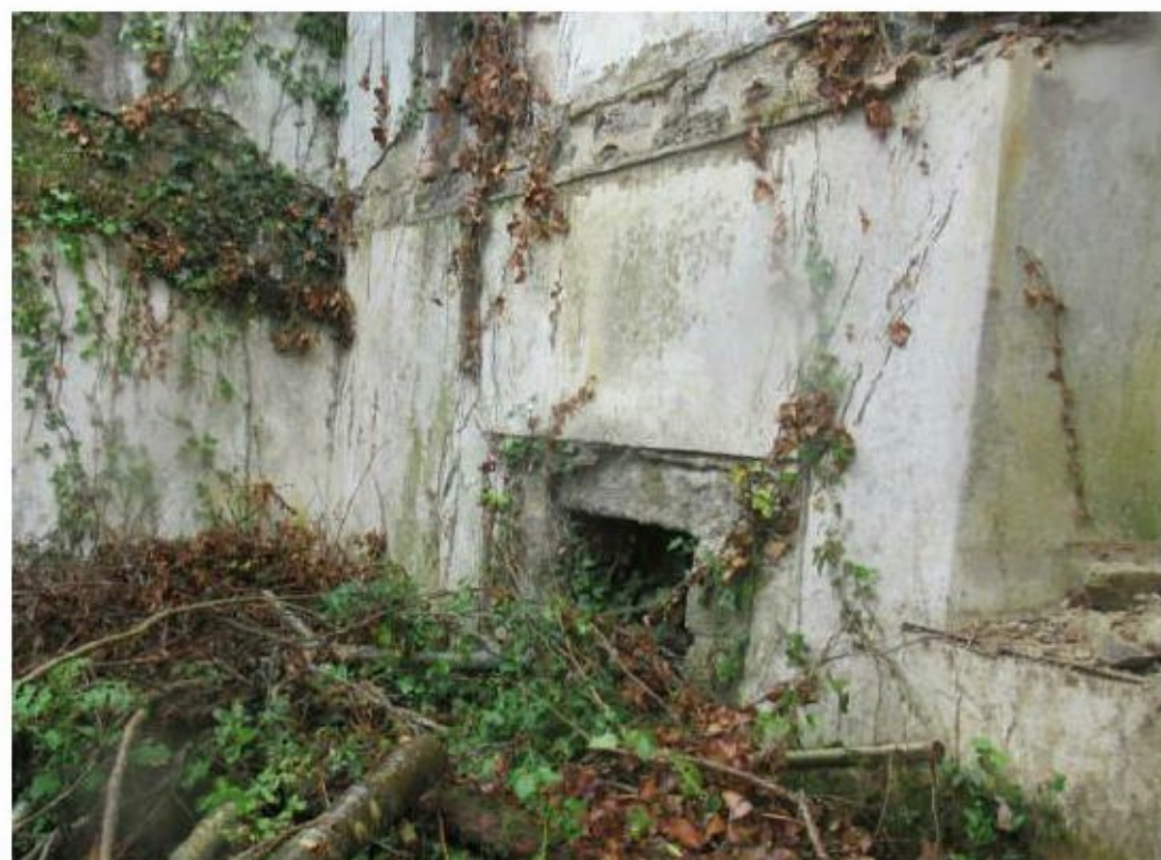
Photo 4: Opening to a fireplace along the western elevation of the cottage
