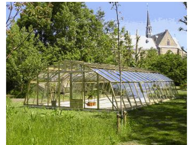
Timber frame dutch greenhouse
