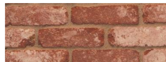
Reclaimed Hertfordshire soft red bricks with half round brick coping
