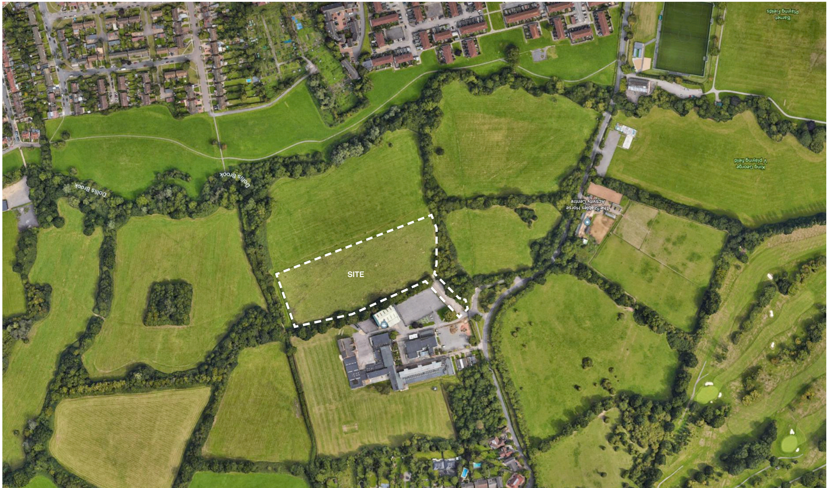
Aerial view of the site
