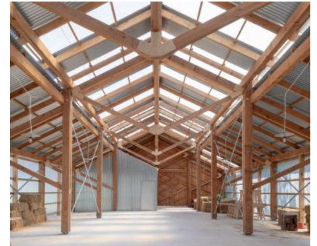
Uninsulated timber frame barn
