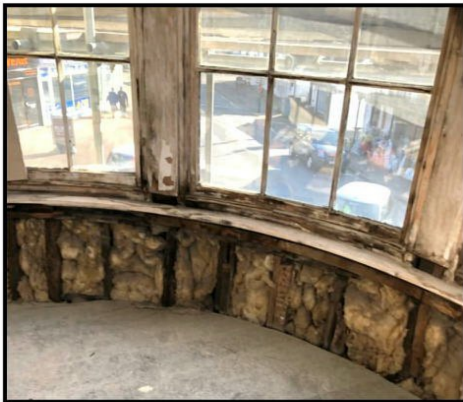
The picture shows the bark timber studwork.
