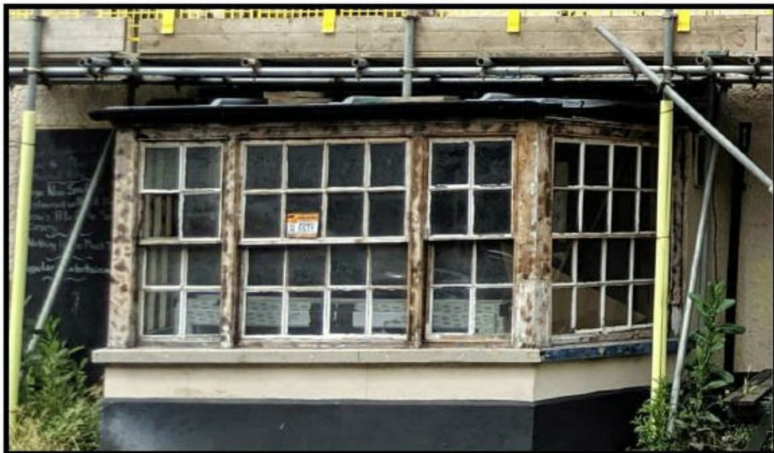
Front bay sash window.
