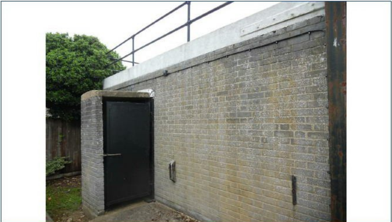
Photo 03 Brickwork walls – gable walls to be constructed to match
