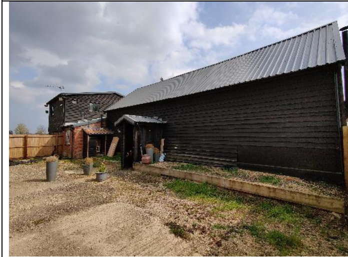
Photo 3 North elevation of barn
