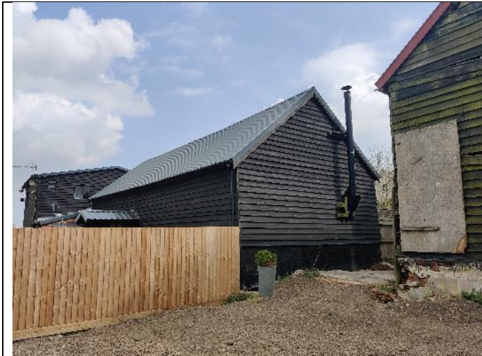
Photo 1 North and west elevation of barn proposed for demolition
