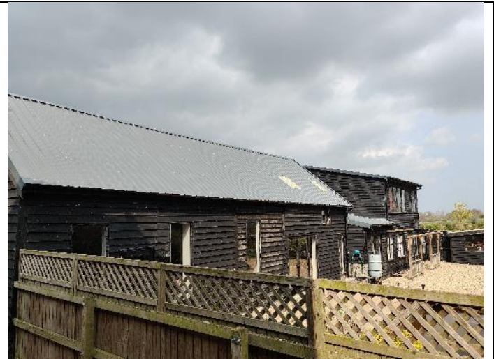
Photo 2 South elevation of barn and hard standing in garden
