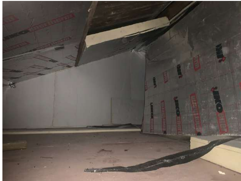
Photograph 7. Gaps around wooden cladding
