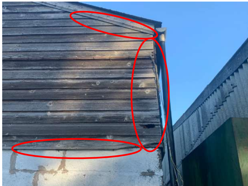
Photograph 7. Gaps around wooden cladding
