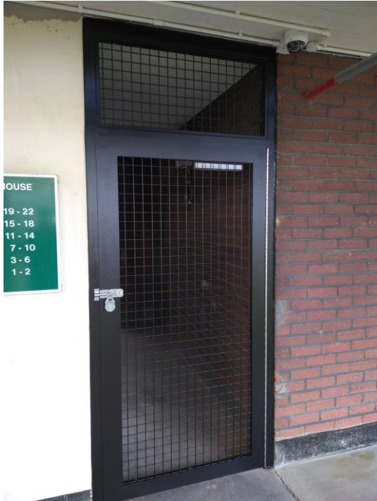
Typical new gate
