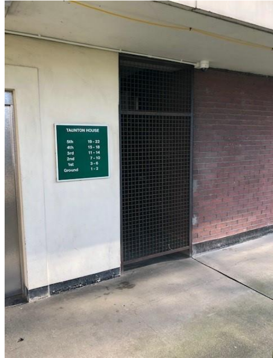
Typical new infill panel
