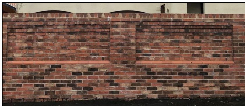
Photo 7. Brick wall detail showing recessed panel and corbelled upper courses.
