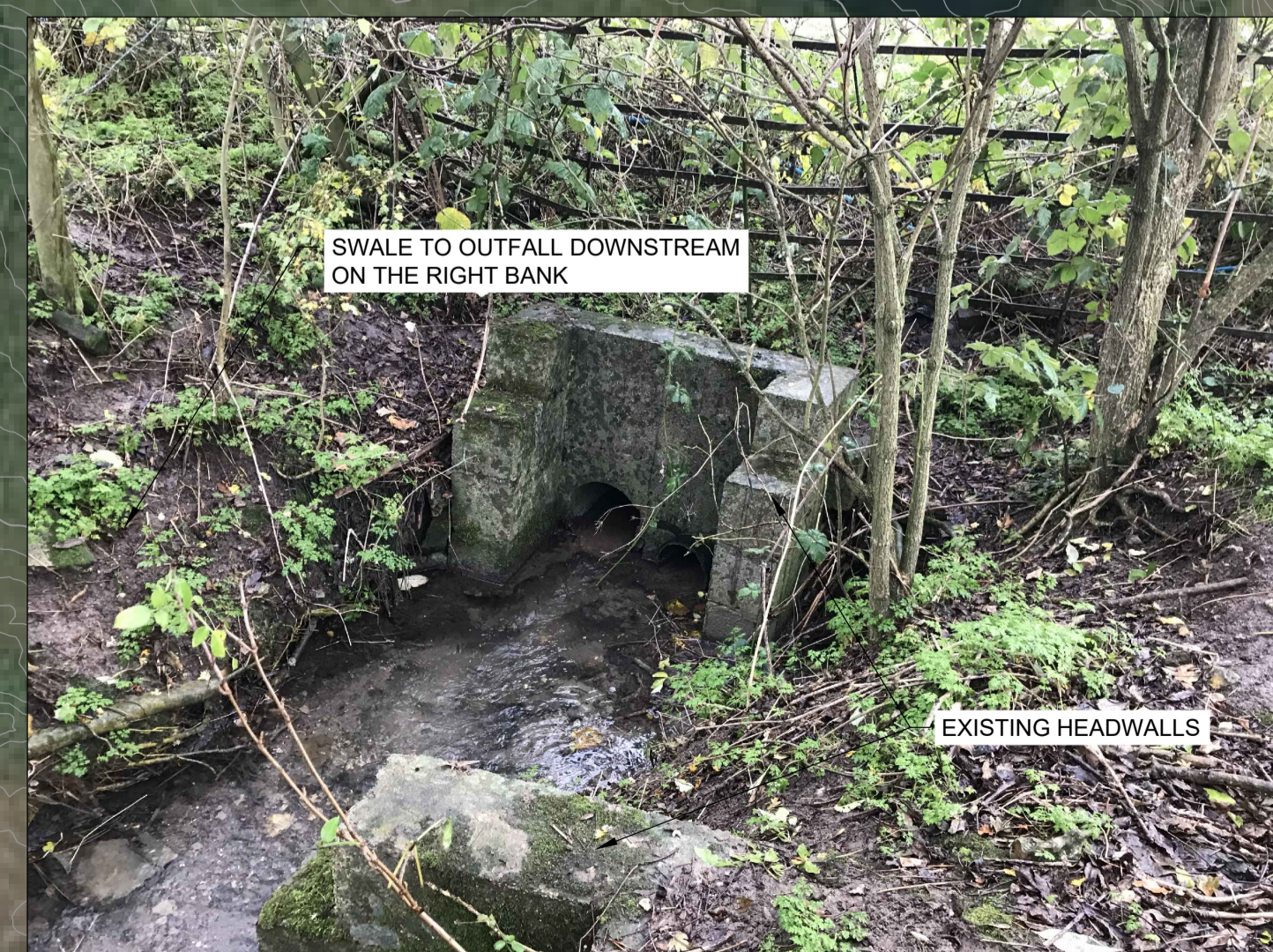
IMAGE 1: EXISTING HEADWALLS AT SWALE OUTFALL
