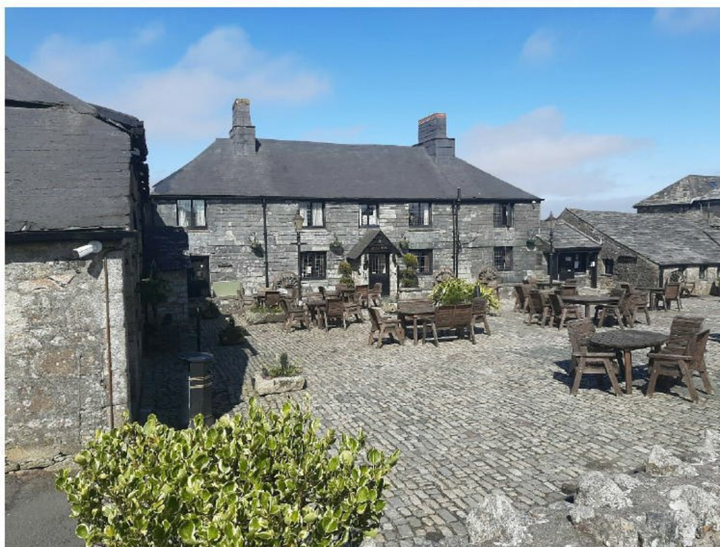
Photo 1: listed building at Jamaica Inn from road.
