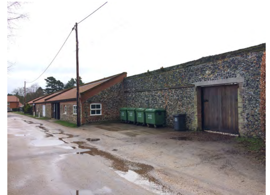
Figure 22: The lean-to buildings attached to the north side of the Walled Garden and the entrance into the garden in the north wall
