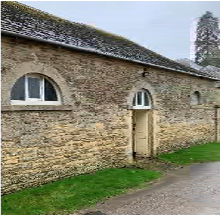
Principal elevation, right hand window to be reinstated.
