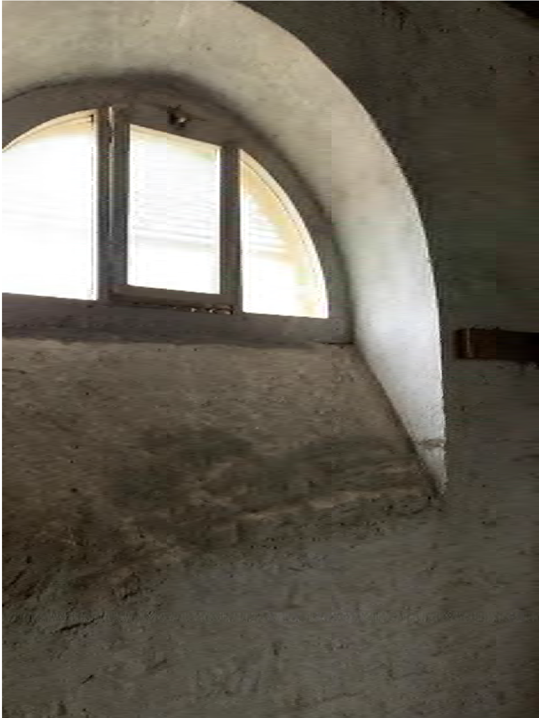
Existing plastered reveals in good order.
