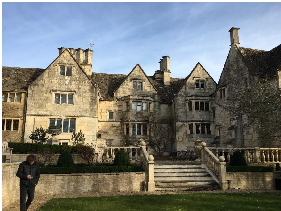
Figure 5: The western, rear, elevations of Court House with relatively recent terraces.
