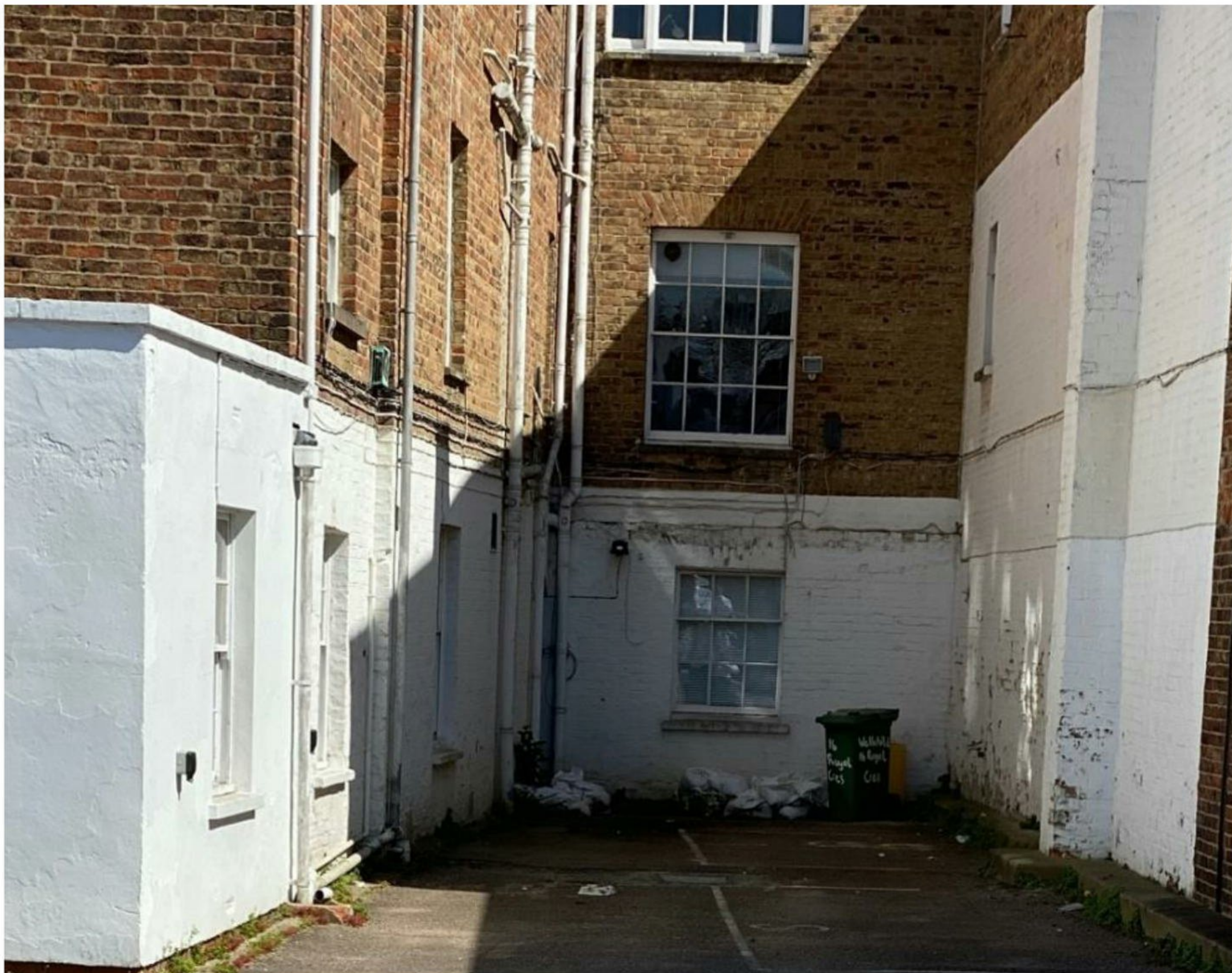
Fig.18 Windows at the rear of No.16 with 3-over-6 sash window at lower ground and 8-over-8 sash at ground floor; note also absence of external steps
