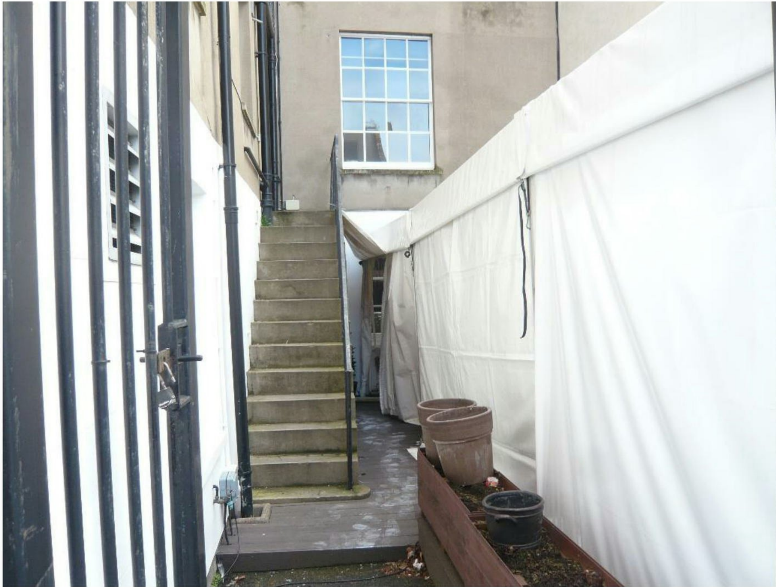
Fig.9 Fire escape staircase to No.12
