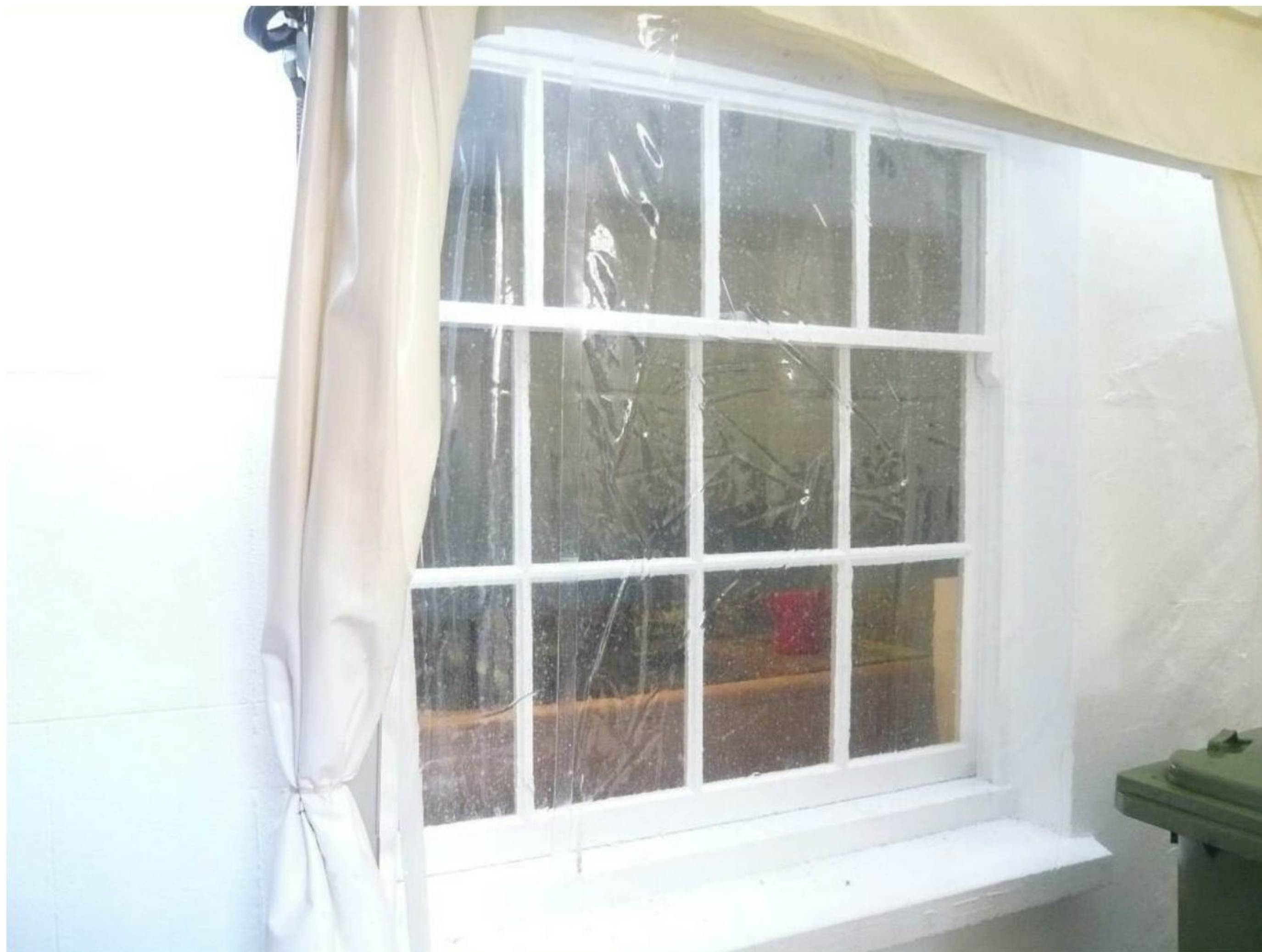
Fig.8 Lower ground floor window of No.12 with horns and concrete sub-cill
