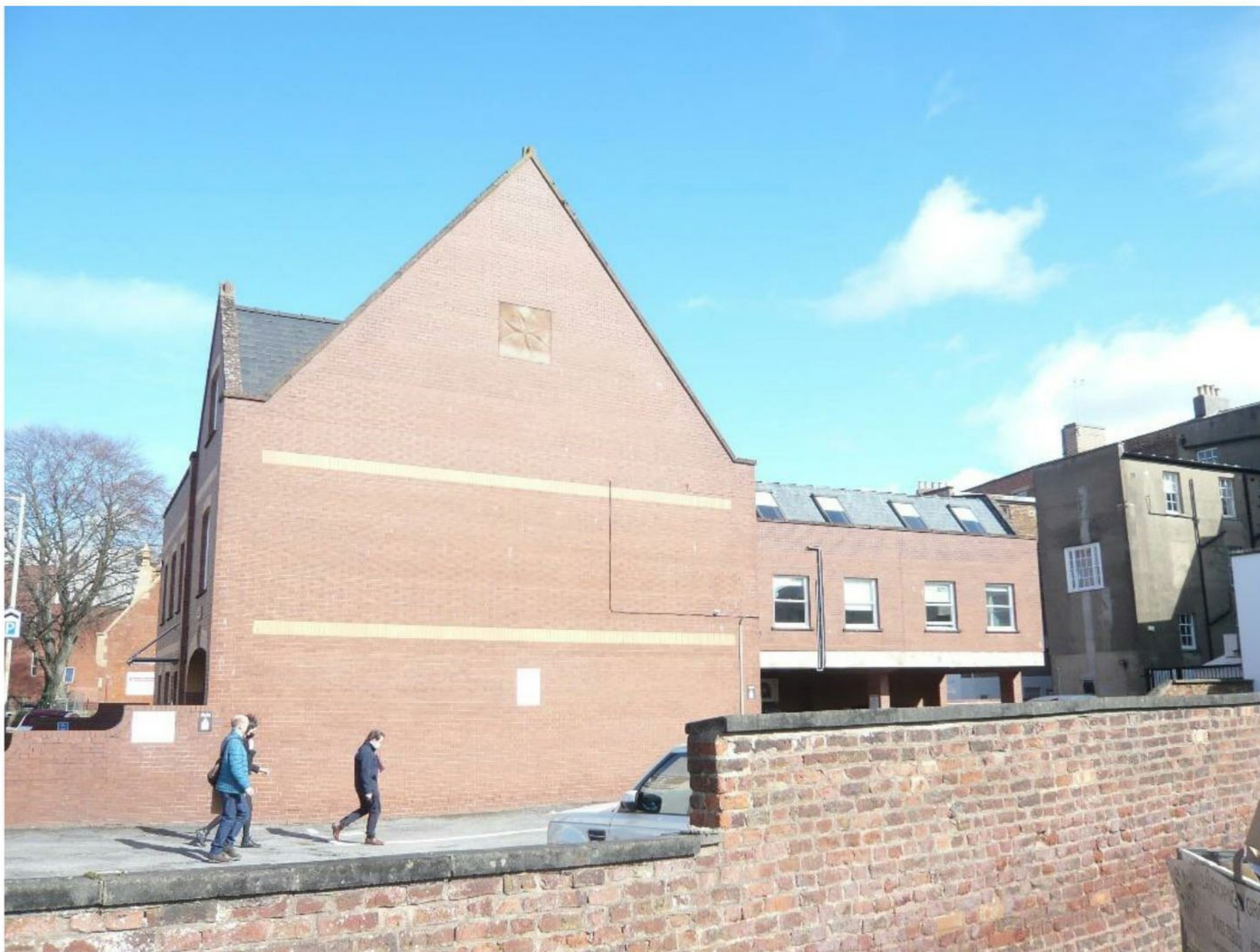
Fig.6 Modern office building to the rear of No.12 as seen from the south
