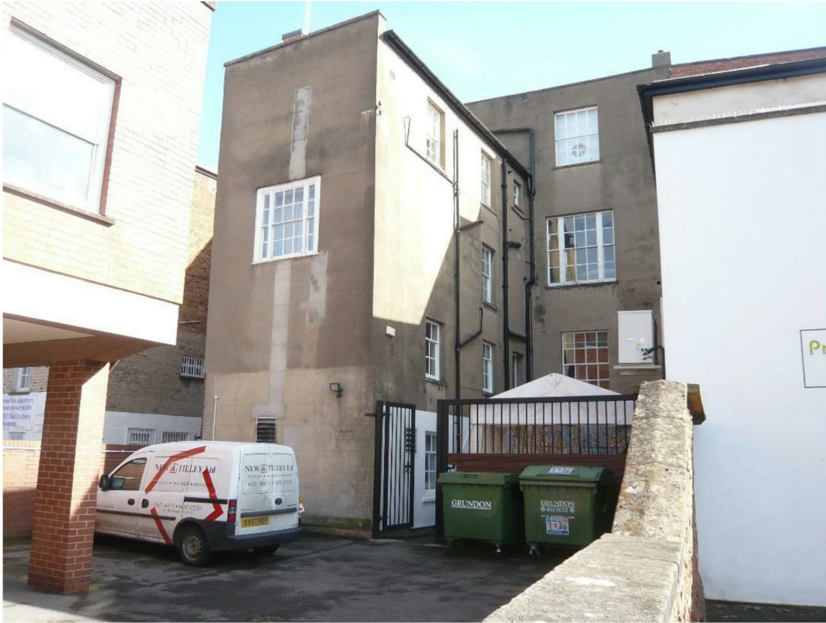
Fig.7 Rear of No.12
