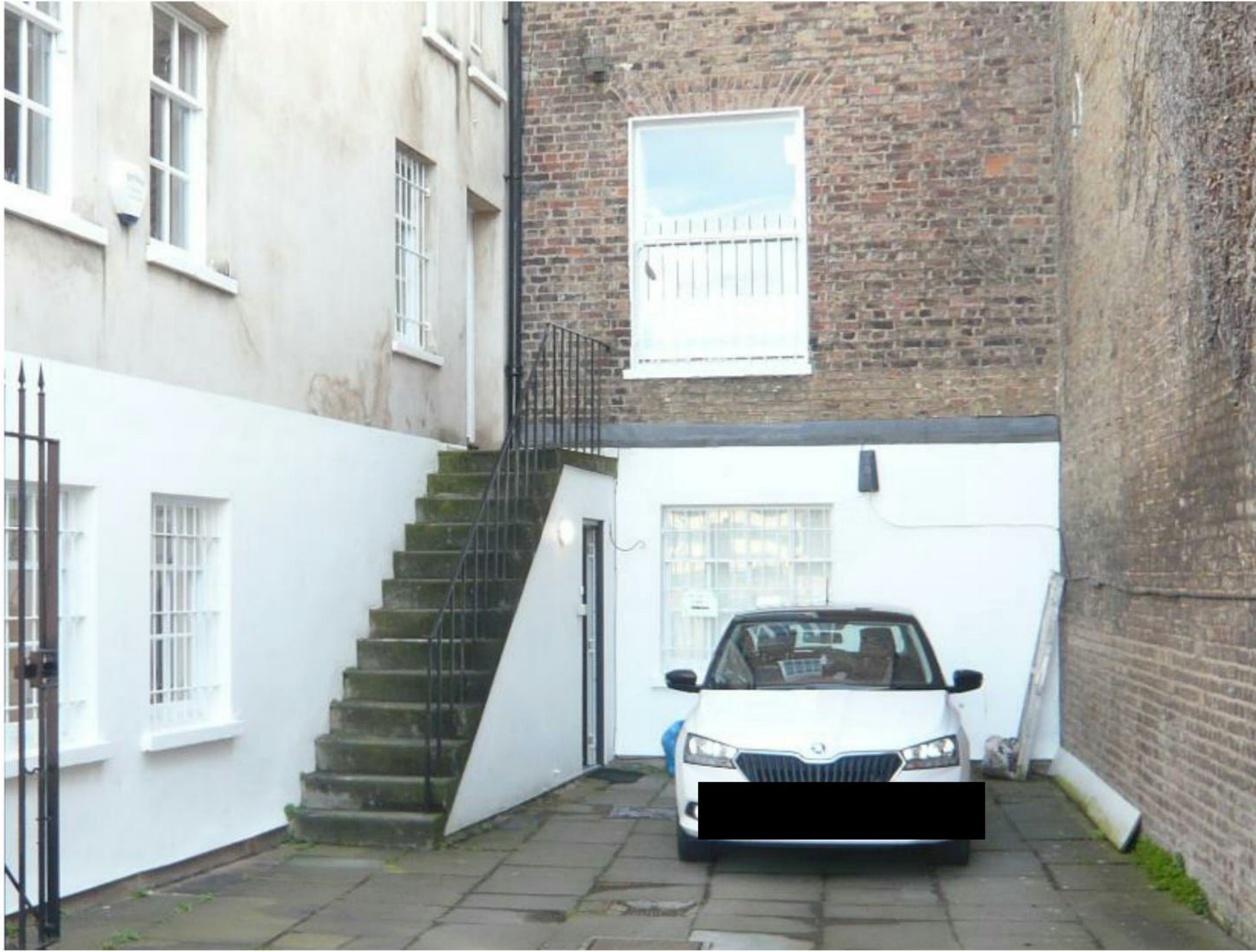
Fig.17 Variation in rear windows within the terrace: The above image is the rear of No.13 with 'wide' 4-over-8 sash window at lower ground floor and single-pane sash at ground floor
