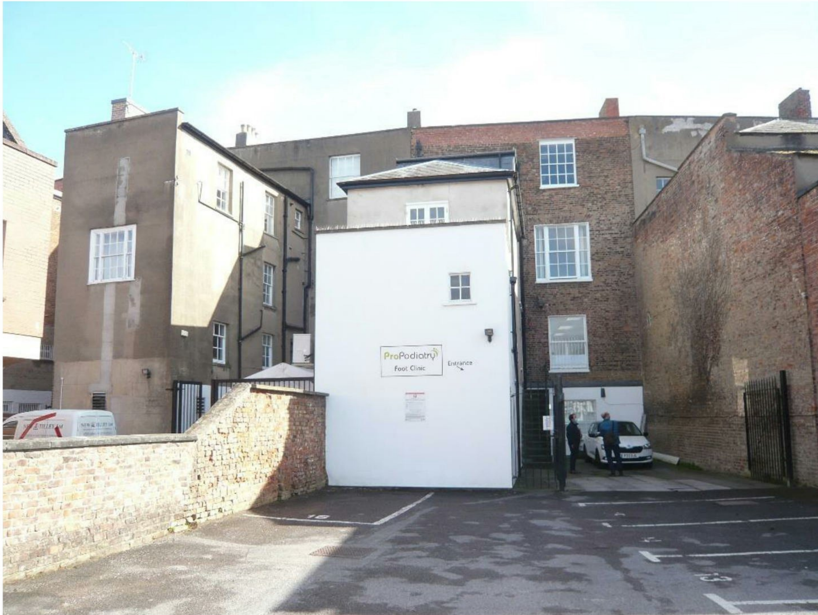
Fig.3 Rear of No.13
