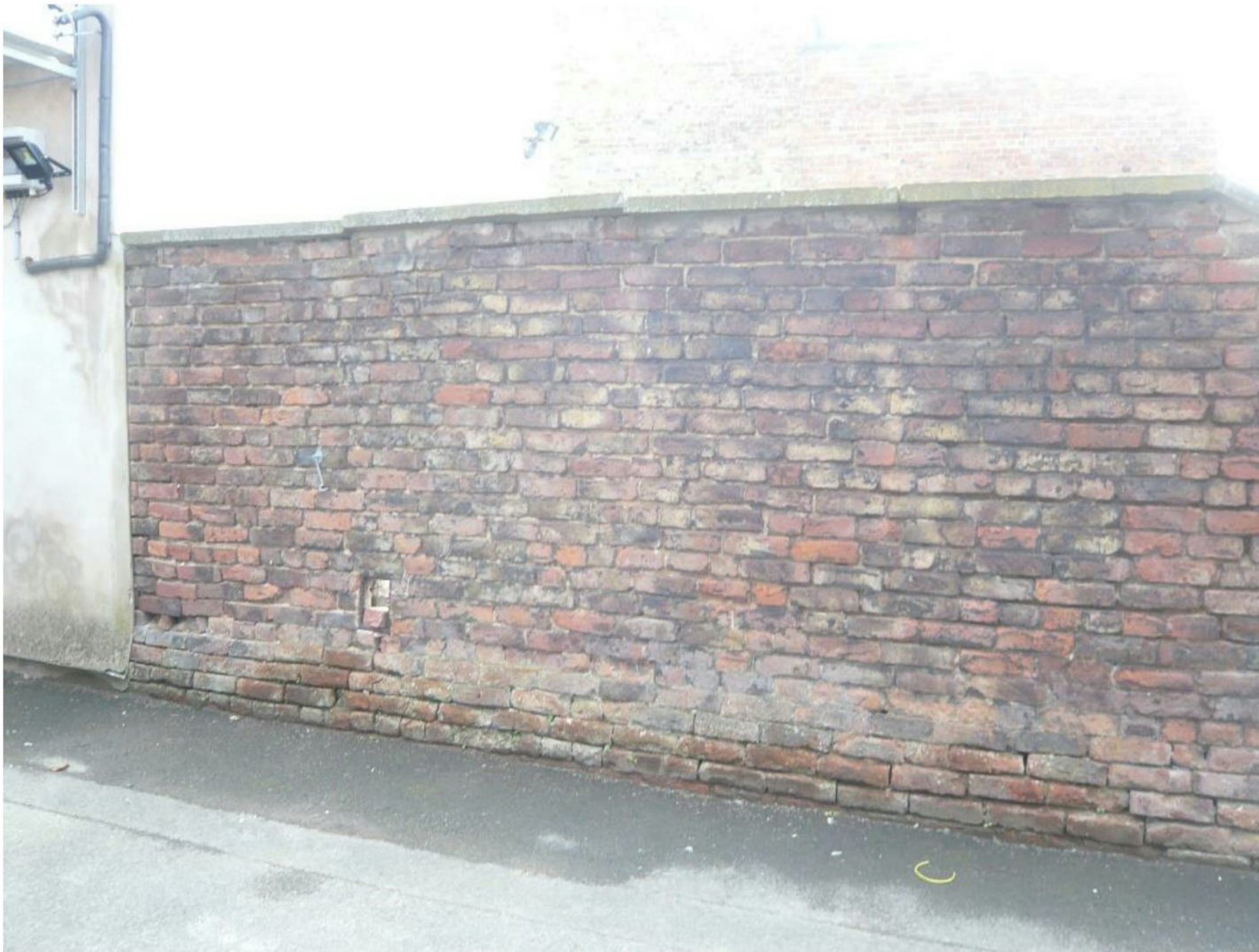
Fig.5 Historic brick boundary wall between the rear plots of Nos.12 & 13
