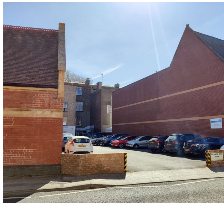
1. View between Crescent Bakery & Royal Mews Building
