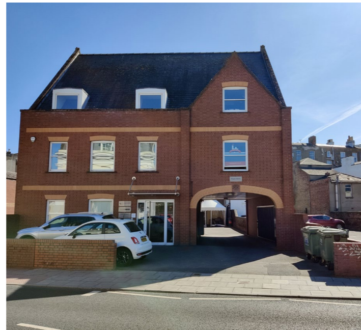
2. View from 77 St George's Place (Grade II Listed)
