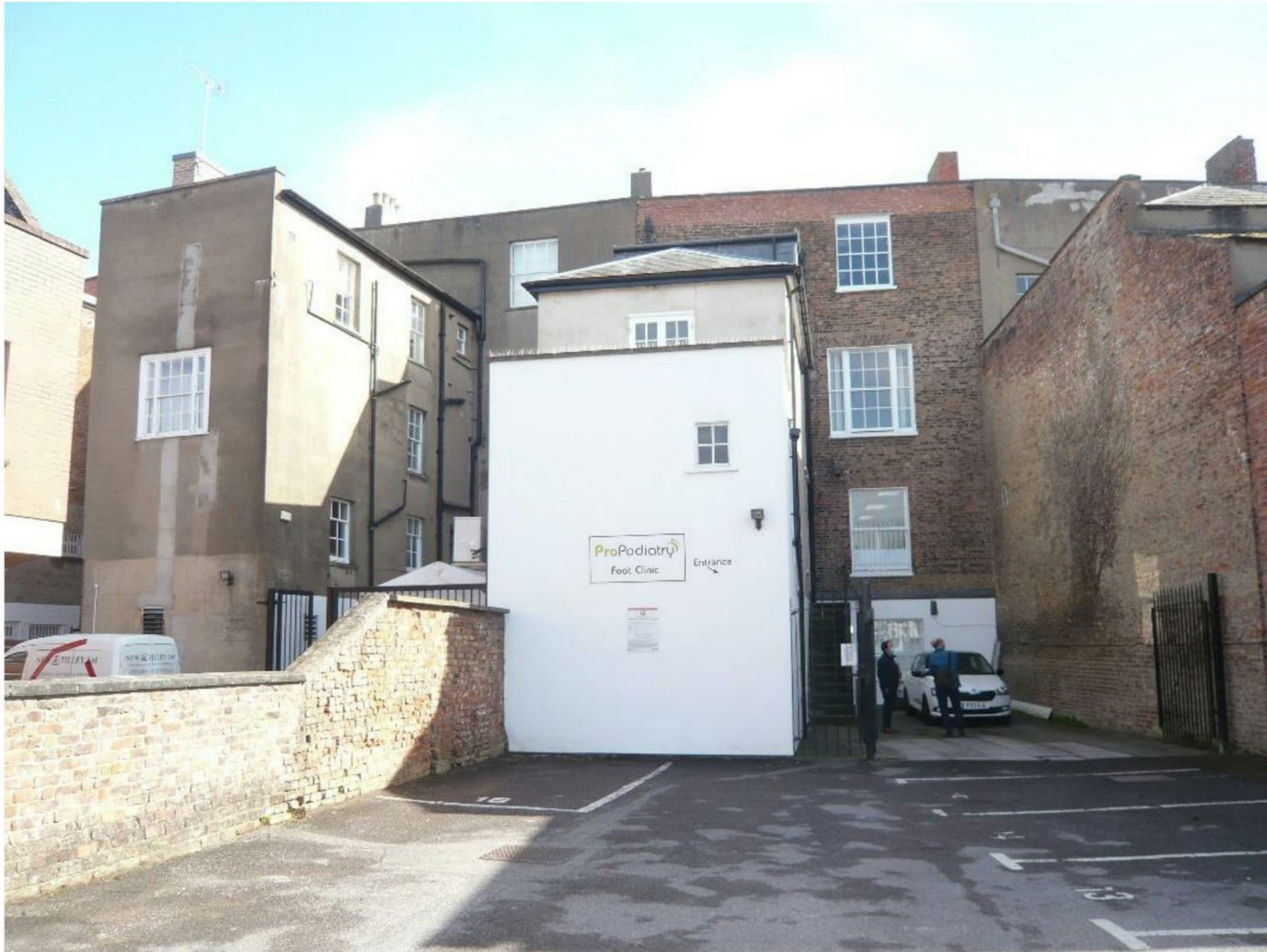
Fig.3 Rear of No.13
