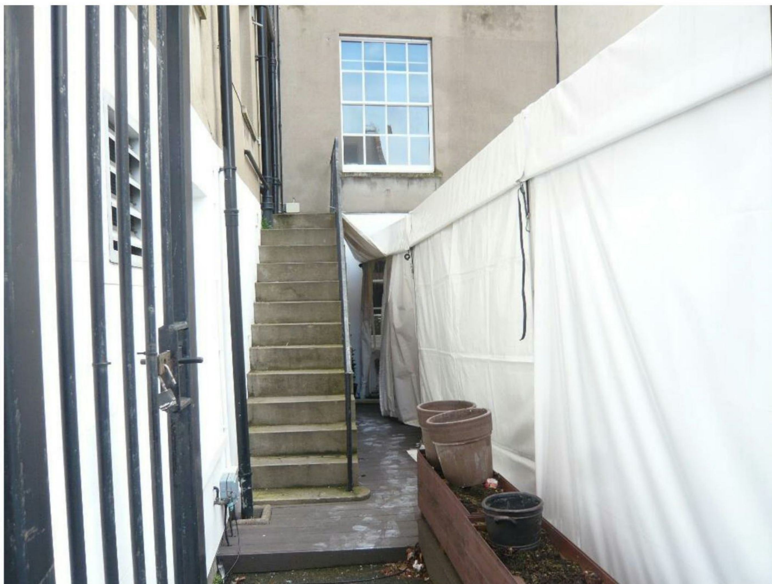
Fig.9 Fire escape staircase to No.12
