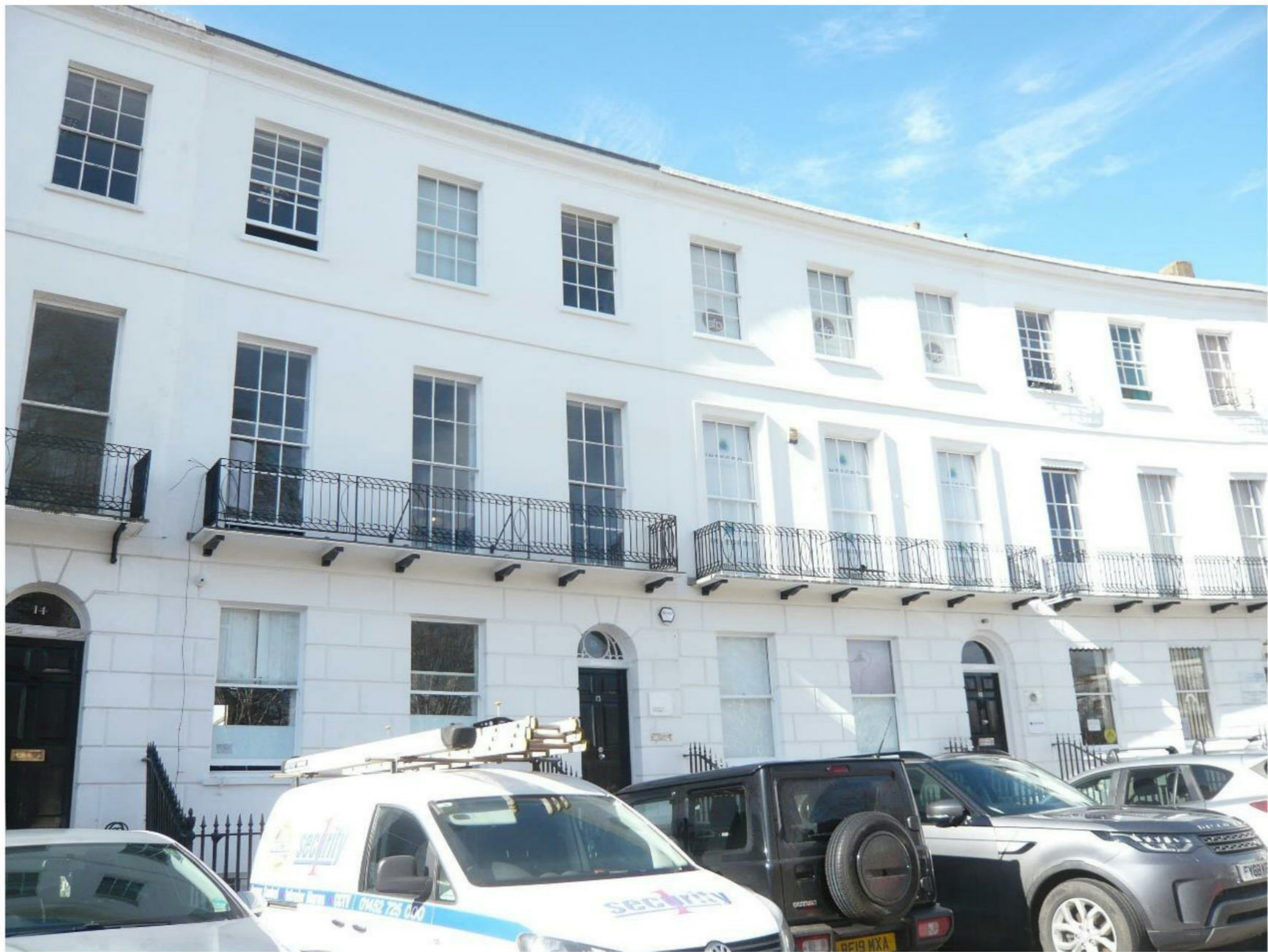
Fig.2 Front of Nos.12 & 13 Royal Crescent
