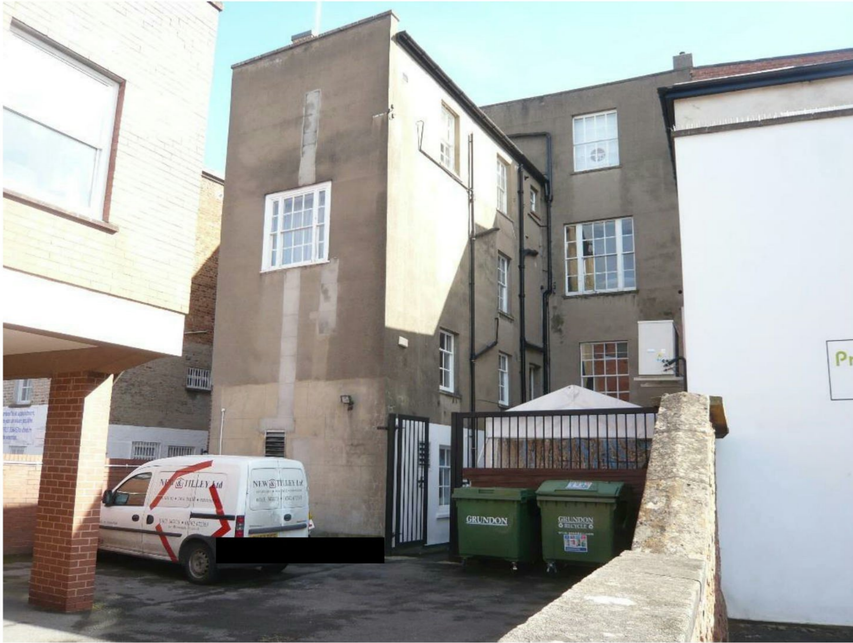
Fig.7 Rear of No.12
