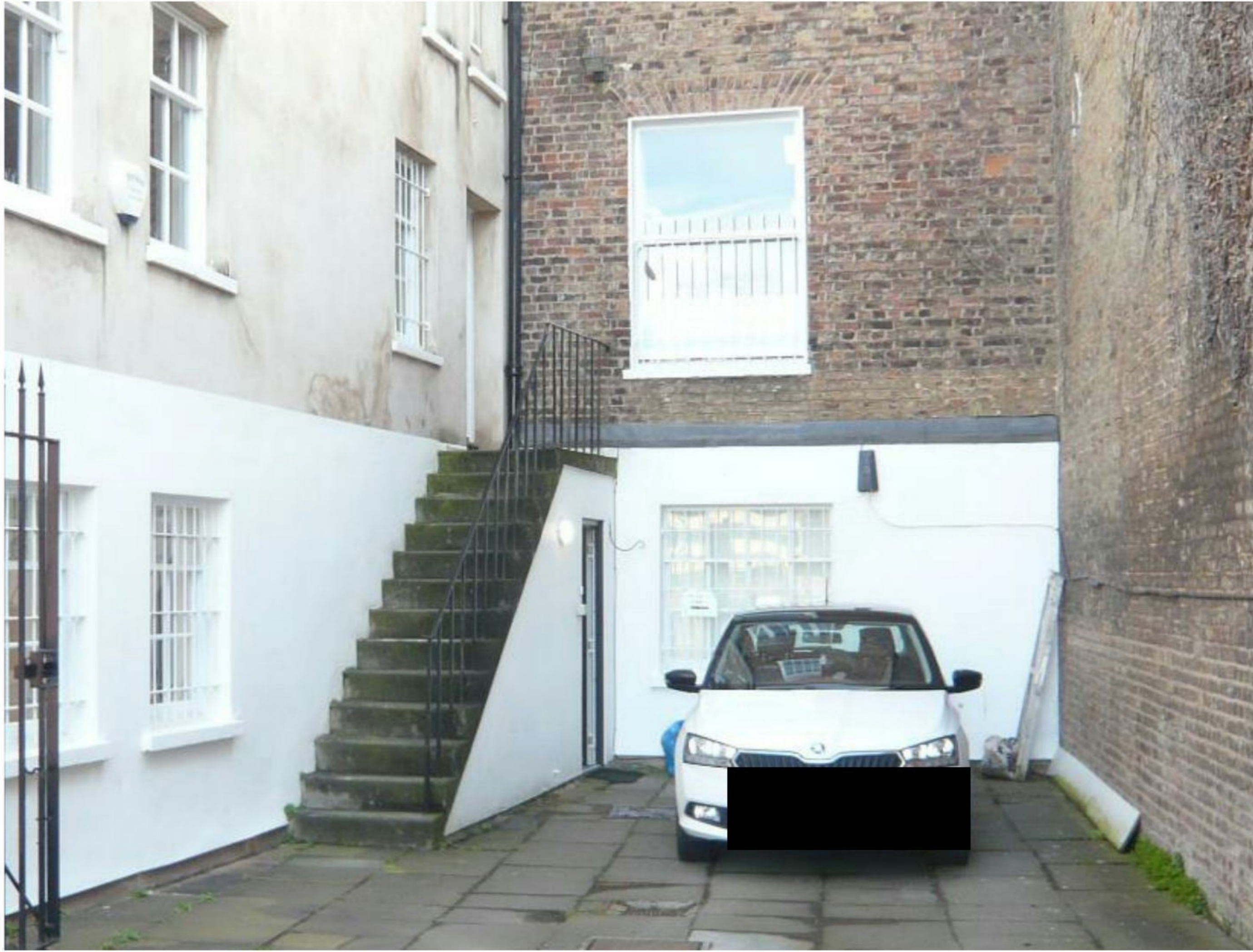
Fig.17 Variation in rear windows within the terrace: The above image is the rear of No.13 with 'wide' 4-over-8 sash window at lower ground floor and single-pane sash at ground floor
