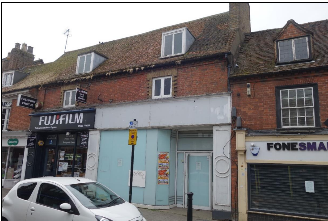
Plate 1: South-facing view of the shop front of 129 – 131 High Street Rickmansworth (Border 2019)
