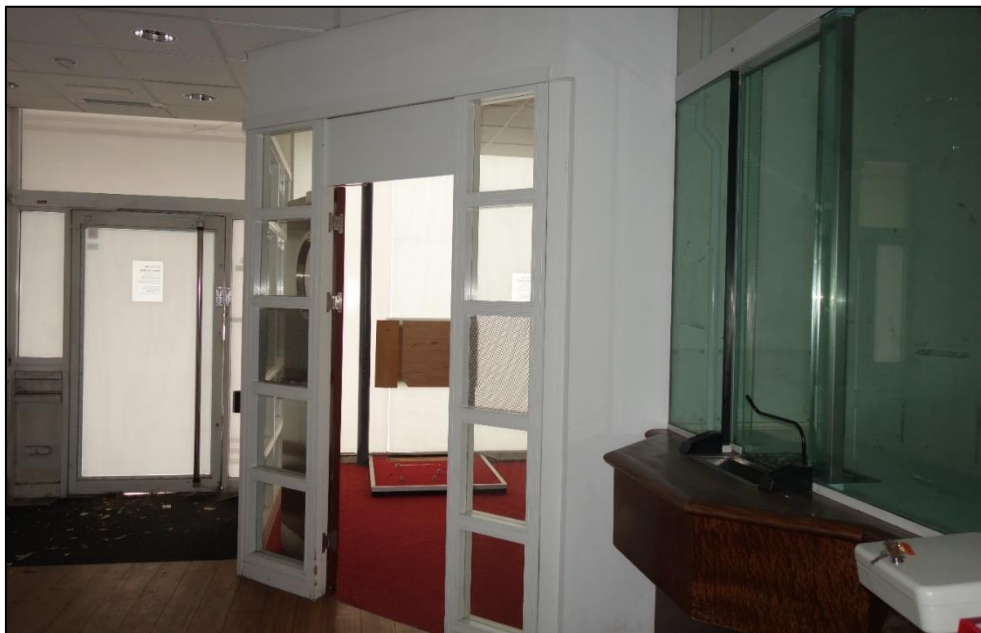
Plate 3: Internal ground floor view of the front of 131 High Street, still with former bank fittings and features (Border 2019)
