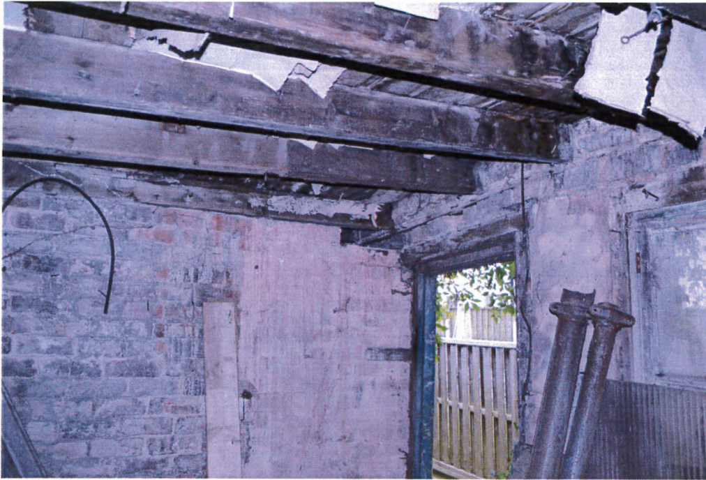
Sloping internal wall in right hand room
