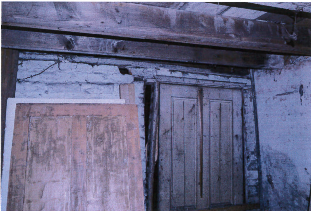
Sloping internal wall in left hand room
