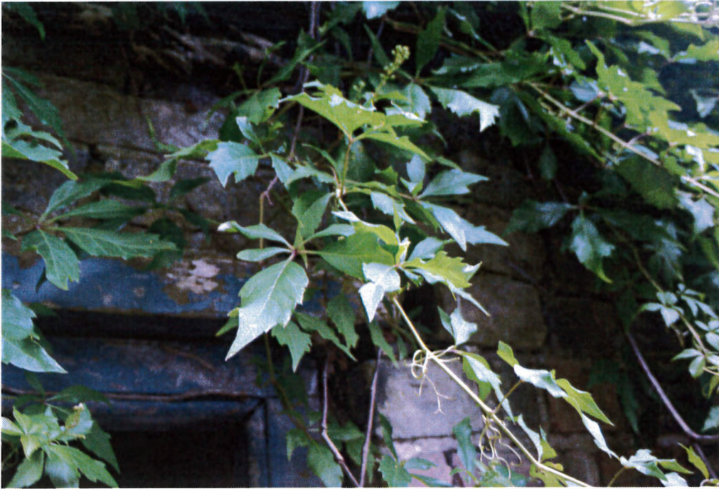
Movement to Front Elevation Doorway
