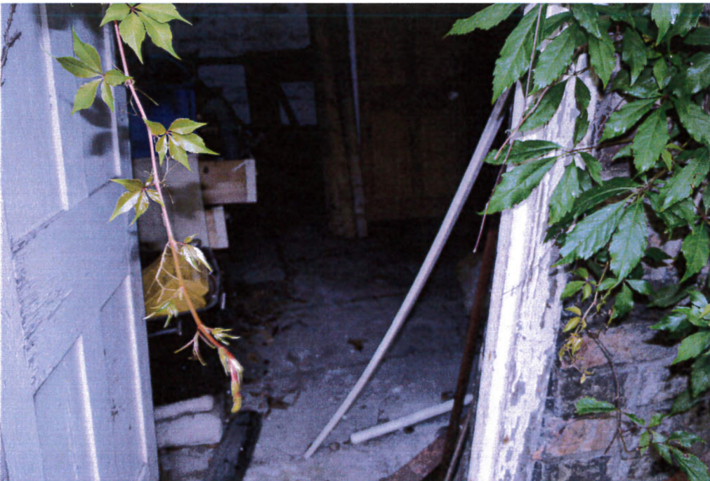
Sloping Floor to Right Hand Room
