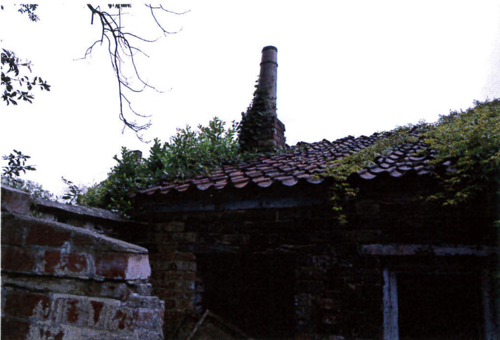
Roof from front
