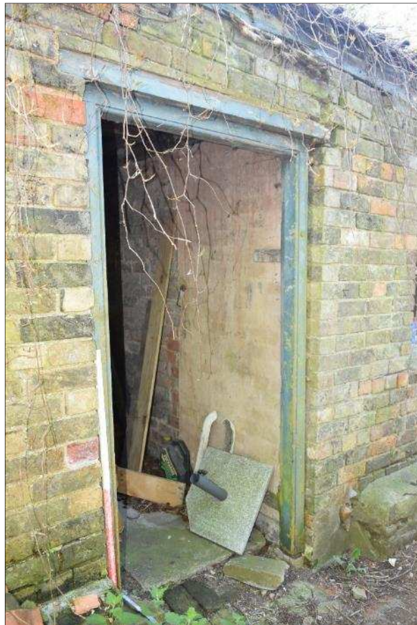
Plate 6 (Shot 7): Door in north elevation living area, looking south-southwest, scale 1m
