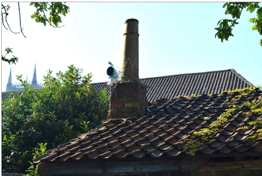
Plate 2 (Shot 11): Chimney stack at east elevation, looking south-southeast
