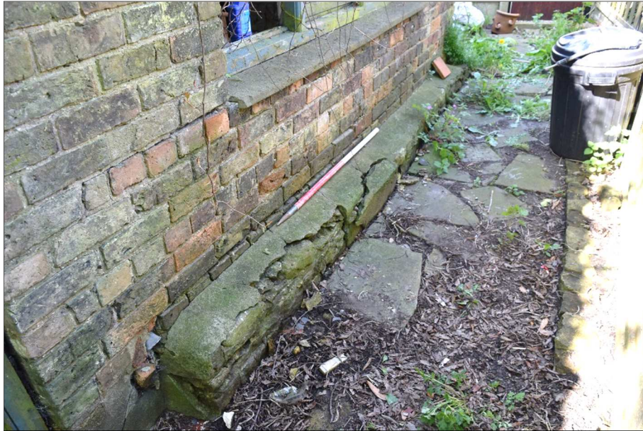
Plate 7 (Shot 25): Plinth on north elevation, looking southwest, scale 1m
