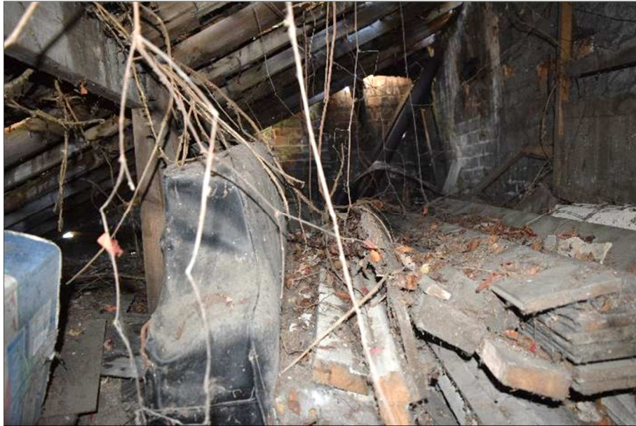
Plate 13 (Shot 21): Loft space, looking east
