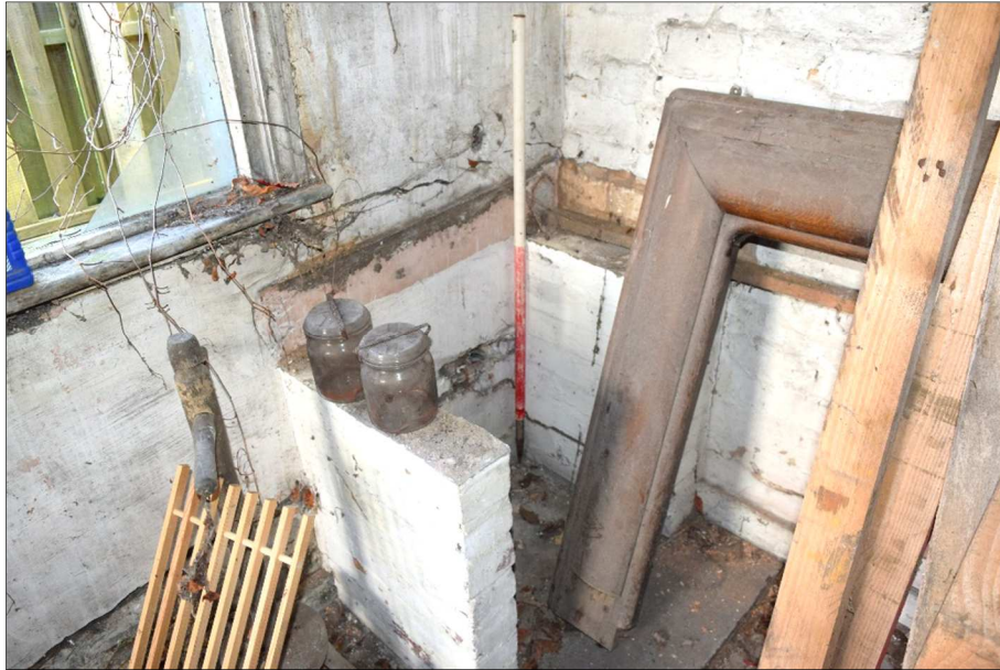
Plate 9 (Shot 14): Stand for wash basin, looking northeast, scale 1m
