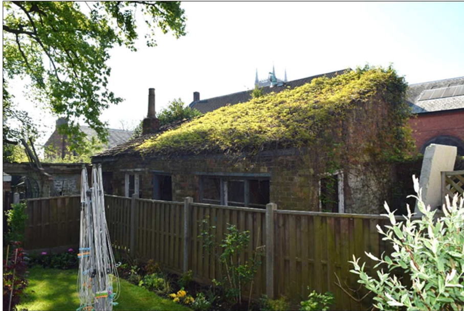
Plate 1 (Shot 2): General view of the building, looking east-southeast
