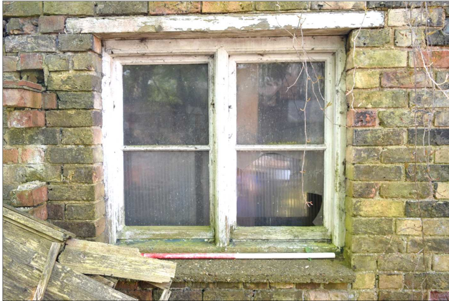
Plate 5 (Shot 9): Window in north elevation living area, looking south, scale 1m
