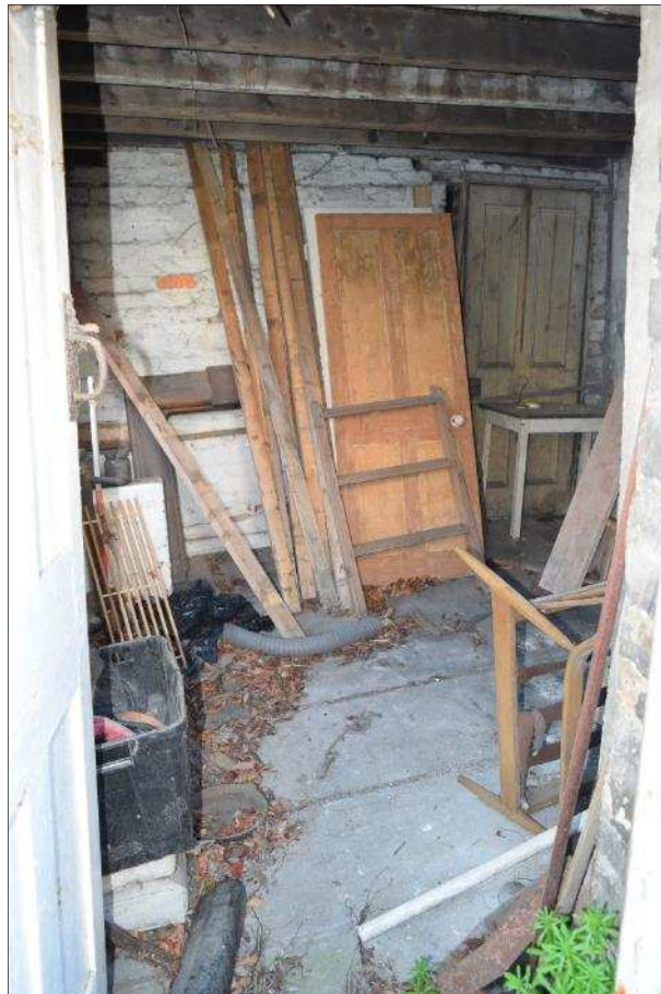
Plate 8 (Shot 13): Scullery interior, looking southeast, scale 1m
