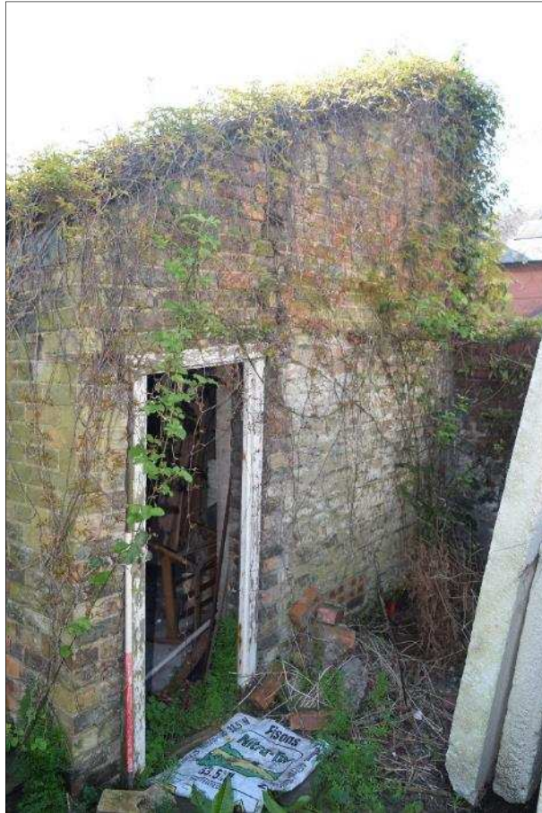
Plate 3 (Shot 4): West elevation, looking southeast, scale 1m
