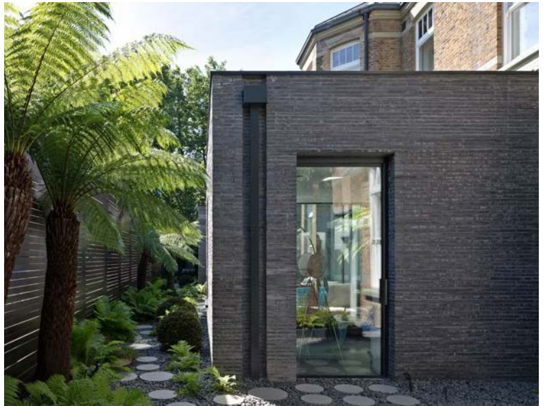
Example of single storey grey brick extension with recessed RWP detail
