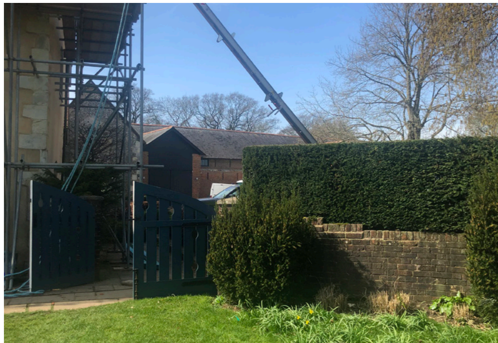
Proposed boiler location (against garden wall of little architectural significance) and concealed from principal elevation view
