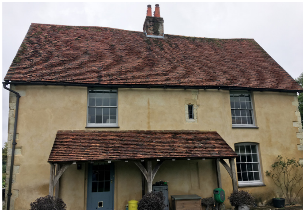
East elevation of Hall Place Main House showing boot room entrance (Existing boiler currently located in Boot Room)
