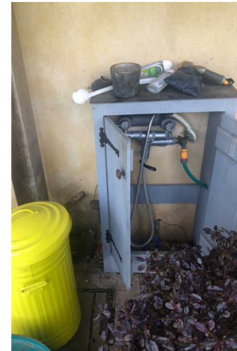
Existing Pipework Housing on East Elevation
