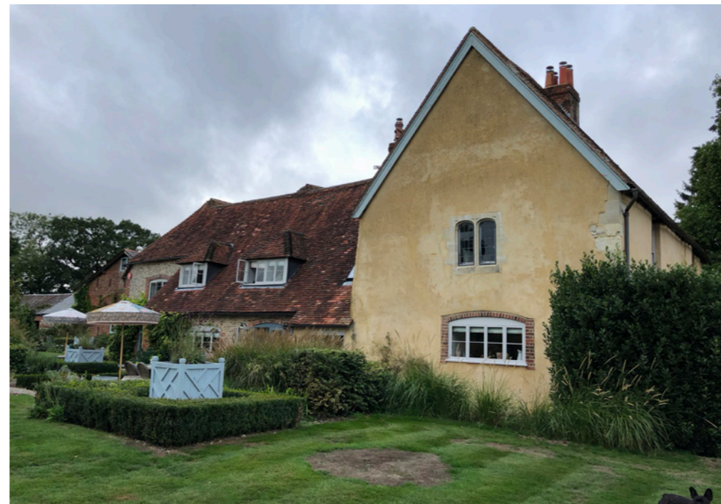
South elevation of Hall Place Main House
