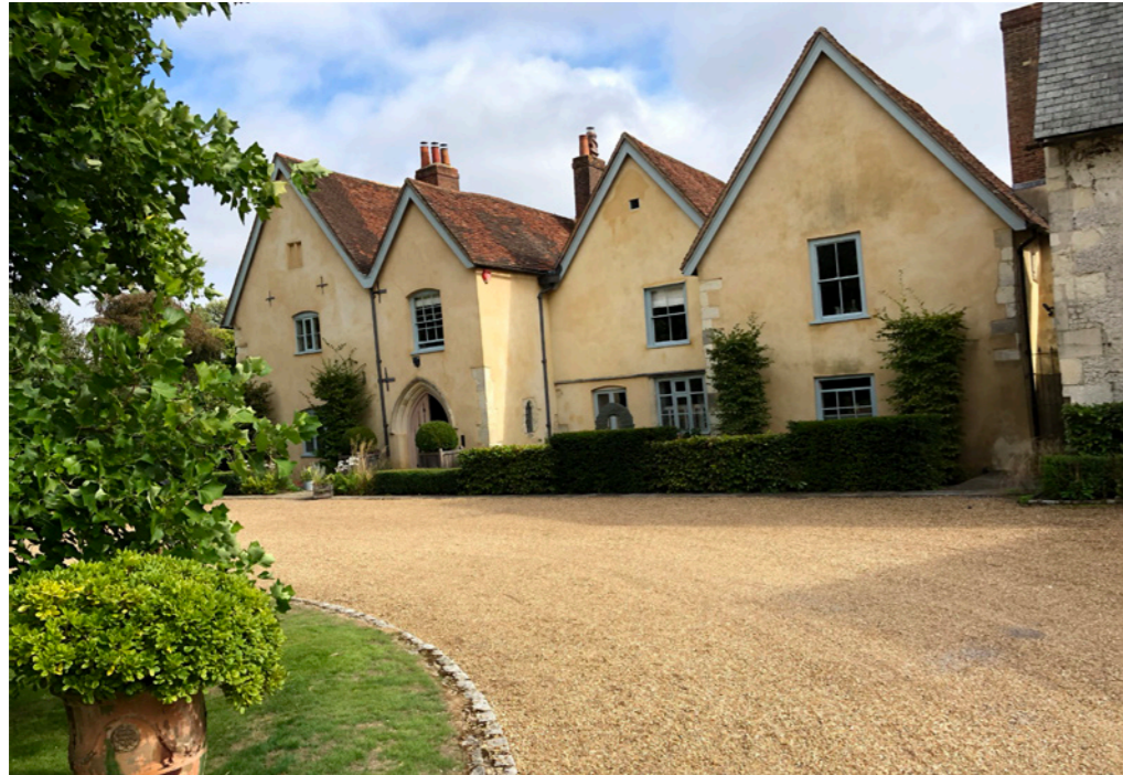
North elevation of Hall Place Farmhouse including entrance to property (Hall Place Chapel to the Right)
