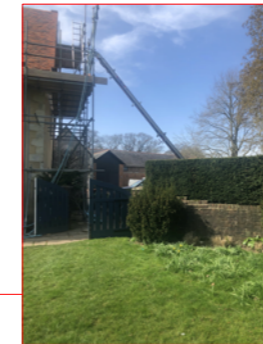
IMAGE SHOWING PROPOSED BOILER LOCATION. SLAB TO BE LOCATED AGAINST BRICK WALL WHICH IS NOT PART OF THE LISTED FABRIC AND IS OF LITTLE SIGNIFICANCE. PROPOSED LOCATION WILL ALSO PREVENT THE BOILER BEING SEEN FROM THE PRIMARY ELEVATION OF THE MAIN HOUSE
