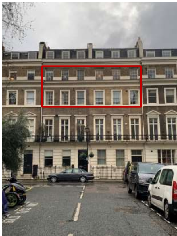
Figure 7 – Nos 31 and 32, now amalgamated into one property Application site ( Flats 3 and 4 are marked with red rectangle).
