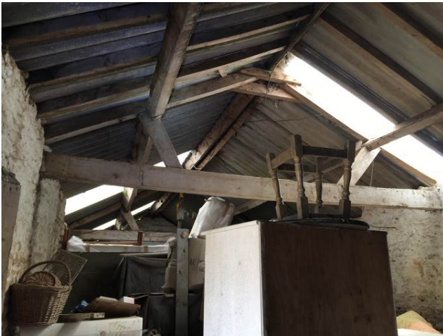
Stable roof interior
