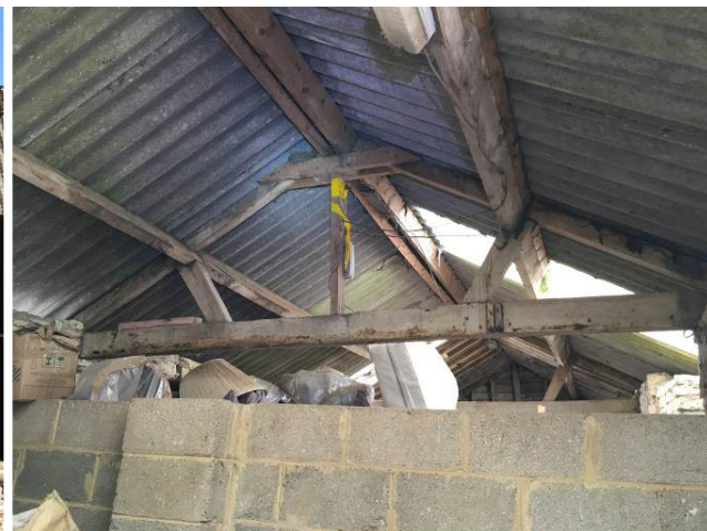
Stable roof interior
