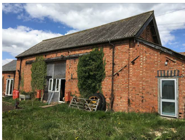
West elevation and south gable
