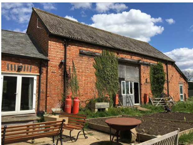
West elevation and north gable
