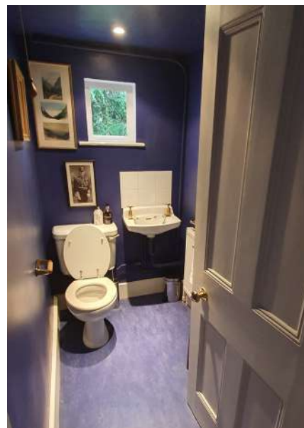
GF existing WC with high-level window
