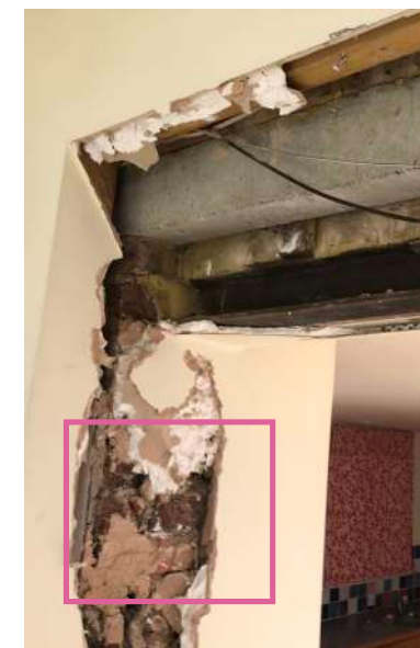
06 Concrete beam cut into wall. New brickwork/concrete/plaster beneath
