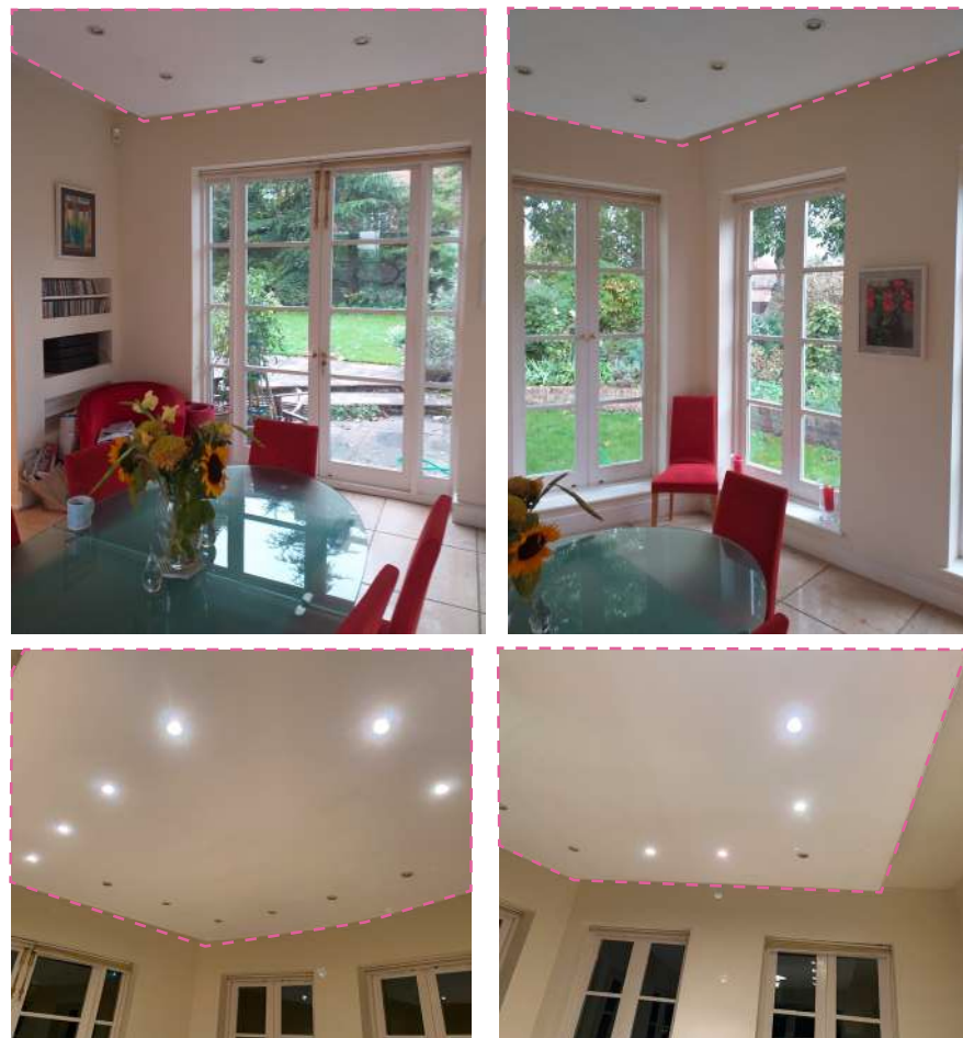
17 Photos of modern suspended ceiling and inset downlights to 1999 Dining-Room extension
