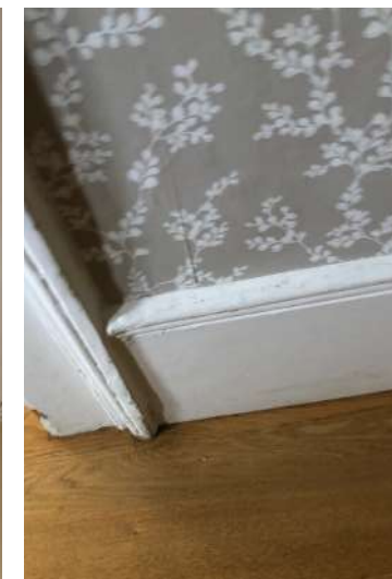
06 Original skirting sections matched
