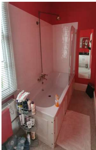
GF existing Bathroom
