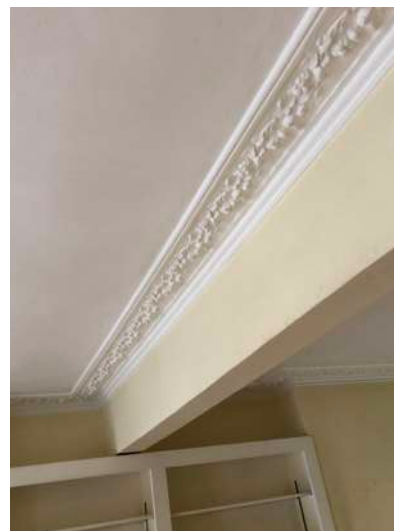
04 Cornicing to Living-Room (not original)
