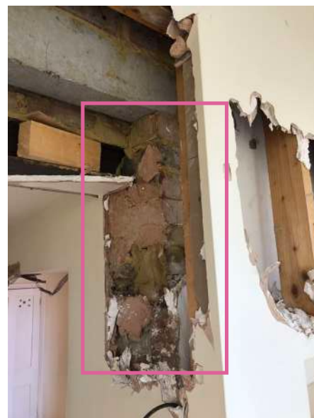
04 Concrete beam installed with modern brickwork pier beneath
