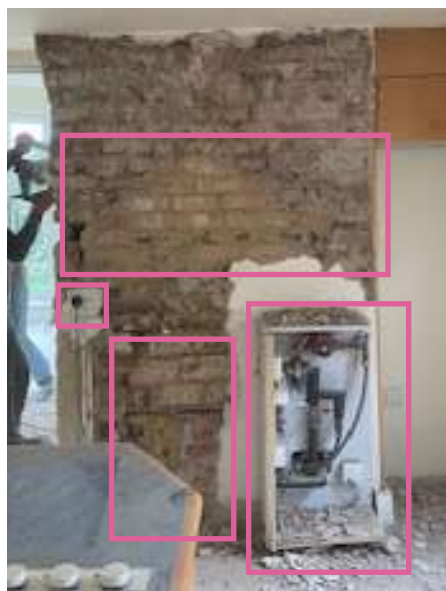
03 Various photographs showing areas of modern brickwork/cement in the original fabric. Also numerous penetrations from modern services.
