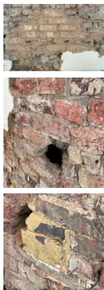
03 Various photographs showing areas of modern brickwork/cement in the original fabric. Also numerous penetrations from modern services.
