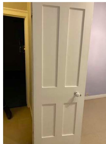
07 Existing timber panelled doors
