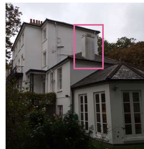
02 Photo showing external chimney stack to be retained.
