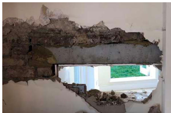
00 Strip-out shows modern concrete beam with modern plaster finish
