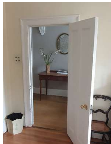
GF Living-Room door to be fixed shut
