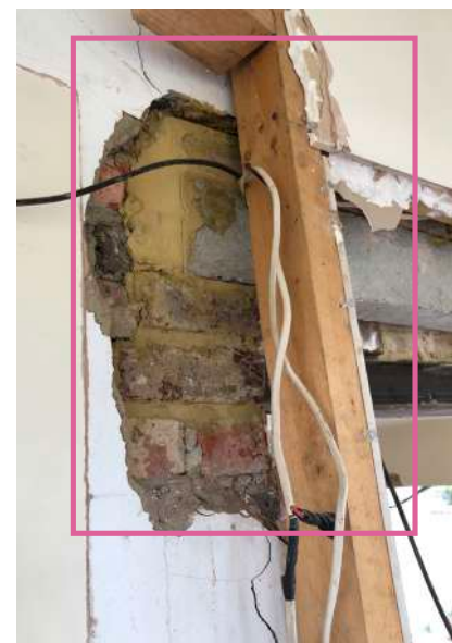
05 Concrete beam installed with modern brickwork beneath
