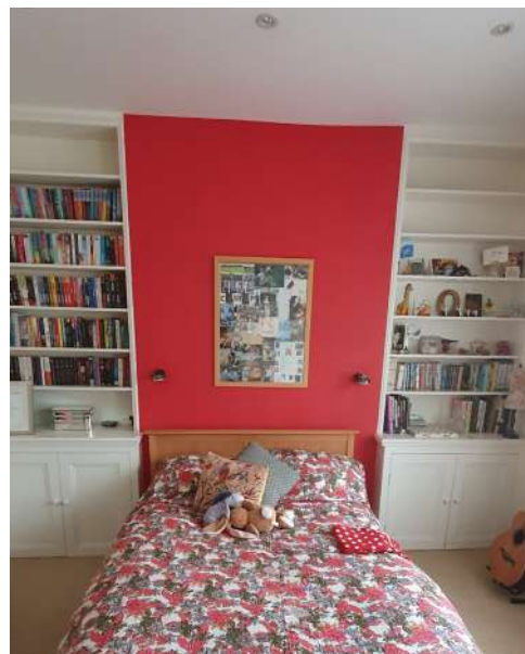
GF existing Bedroom with blocked-up chimney-breast
