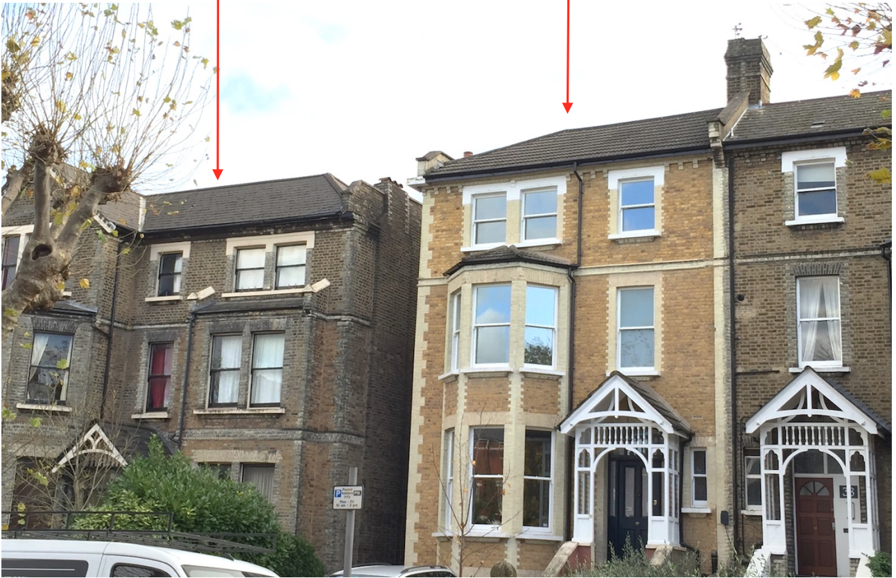
View from Christchurch Avenue
