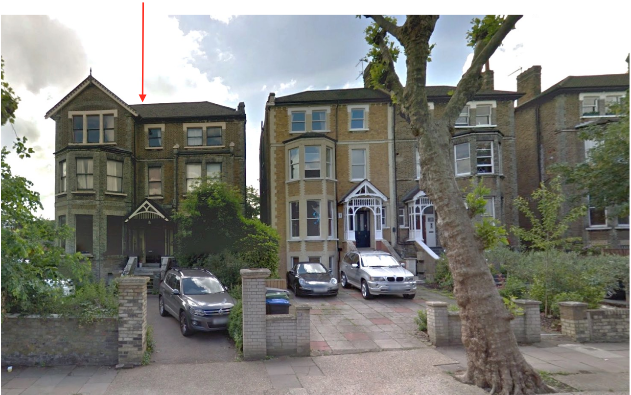
Front view from Christchurch Avenue
