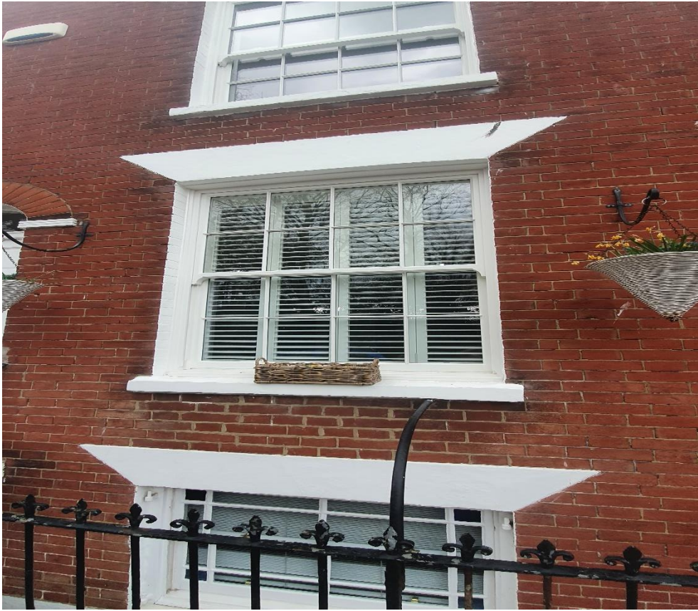
Photograph of proposed new timber sash windows
