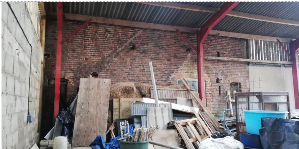
West Elevation (from inside adjacent barn)
