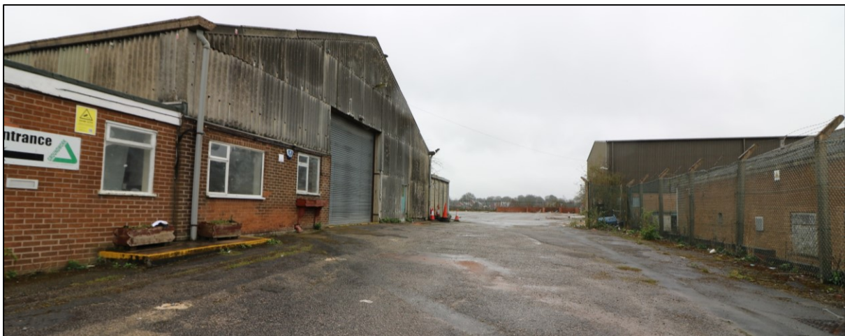
Figure 3: View across the Site looking southwest
