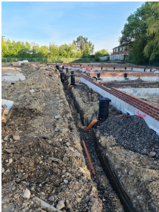
Photographs showing the construction of private (L) and adoptable (R) drainage runs confirm drainage was laid in accordance with Building Regulations Document H, and to Sewers For Adoption standards. Also per the detailed construction design shown on Carley Daines and Partners drawings.
