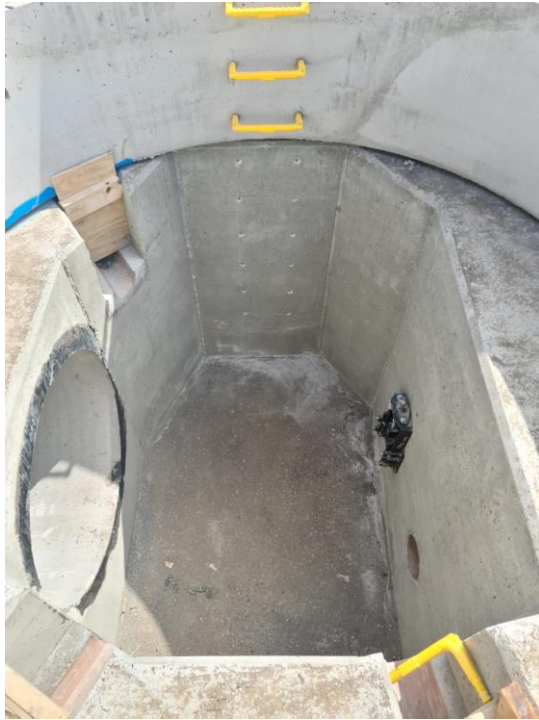
Internal and external photographs chamber S7, containing the Hydro-Brake. Constructed in accordance with Carley Daines and Partners drawings and Hydro International.
