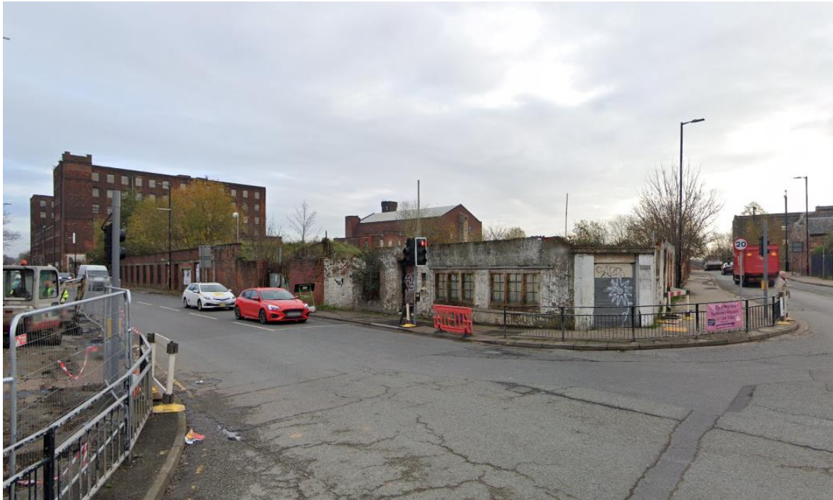
Figure 11: Existing Corner Structure
