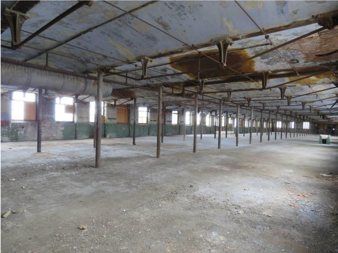
Figure 39 – The unaltered fifth floor of the main mill building, parallel with the Aston Canal. This view illustrates the original open-plan design of each floor level, and retains terracotta quarry tile flooring and 1930s paint scheme.
