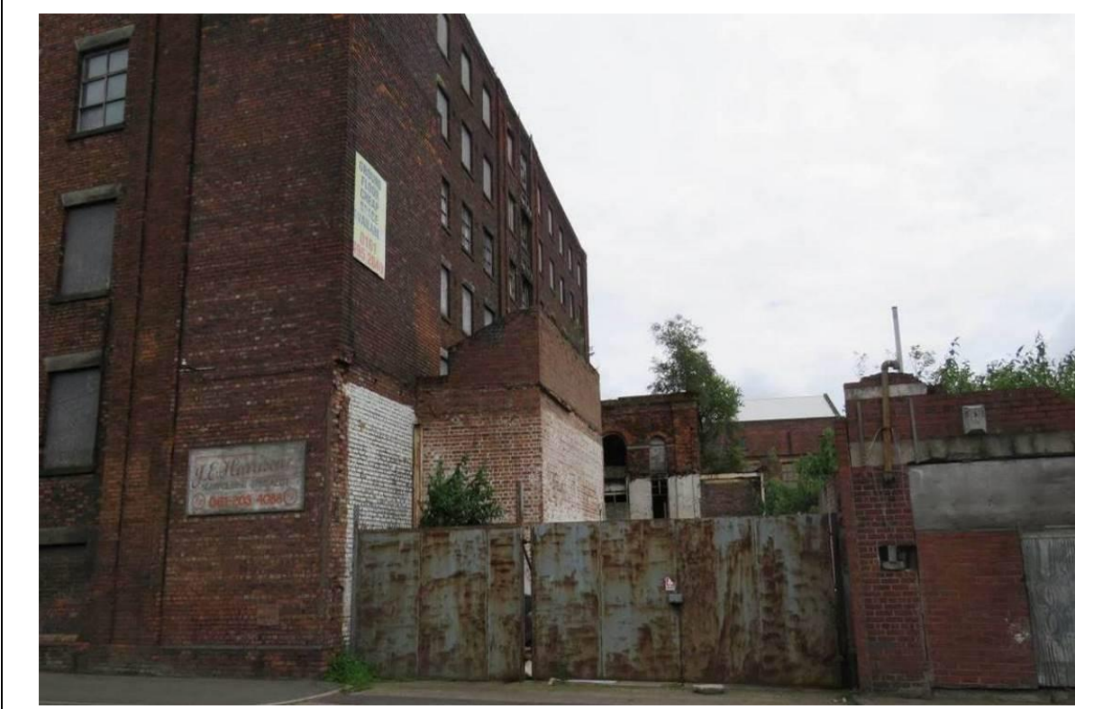
Figure 32 – A view of the former location of the original mill chimney. This view shows the original engine house to the rear, denoted here by two round-headed windows. To the left of the view is the tall, brick dust chute.
