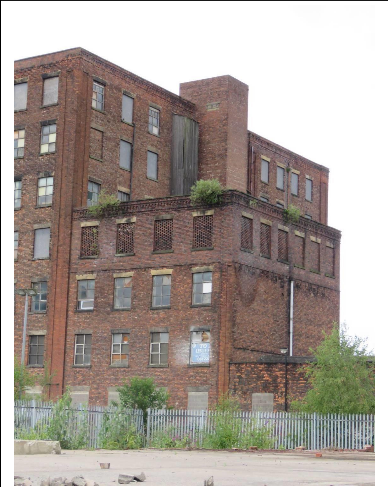
Figure 30 – A closer view of the east wing and 1844 waste house, showing the added c1920s top floor.
