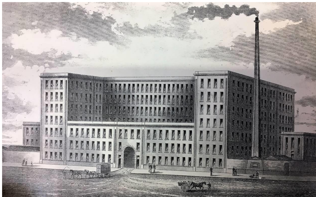
Figure 4 – An 1893 etching of the principal north front of Brunswick Mill as seen from Bradford Road. To the left can be seen the Waste House, whilst to the right is the engine house and chimney. Note the original form of the projecting cornice around all eaves of the buildings.
