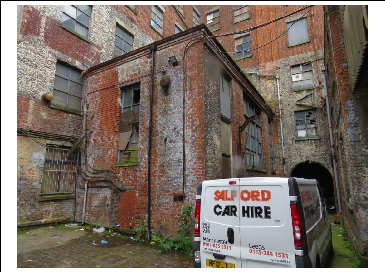
Figure 15 – The remains of the simple and functional 1908 transforming station as seen in 2016.
