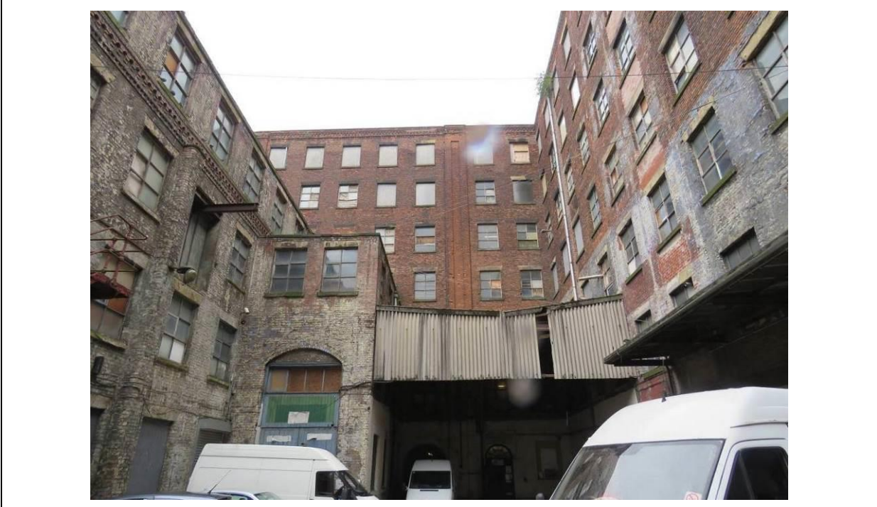
Figure 51 – Looking east across the internal courtyard, showing the entrance block to the left, and main mill building to the right. The three-storey building in the left-hand corner was built in the c1880s, and heightened by one storey in the 1920s.
