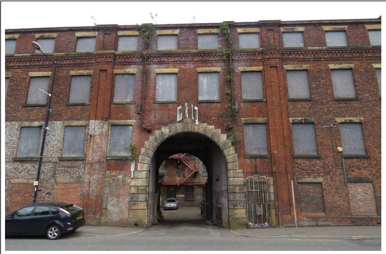
Figure 26 – The north front of the mill, showing the rusticated entrance gateway and two pedestrian portals either side, and blocked ground floor windows. The top floor level was added during the 1920s.
