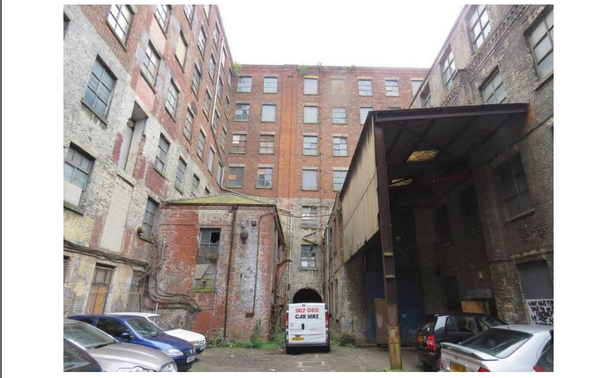
Figure 52 – Looking west across the internal courtyard.
