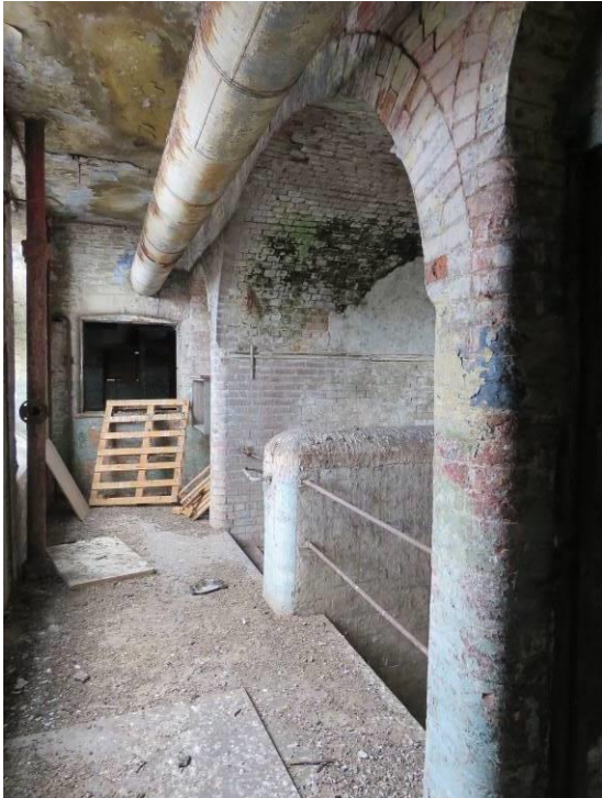
Figure 49 – The top (seventh) floor staircase hall of the east wing, showing the staircase's termination in the form of an unusual domed, semi-circle.
