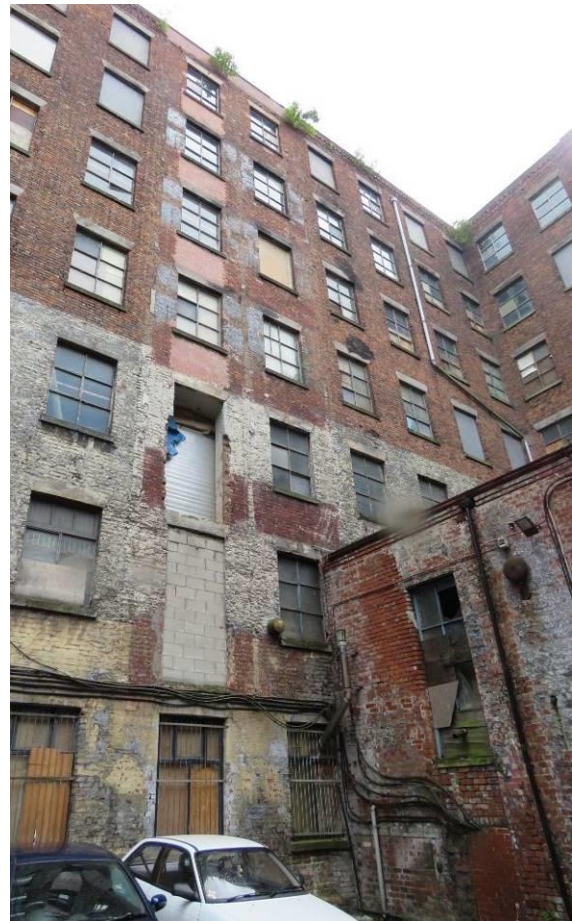
Figure 12 –The same view as seen in 2016, showing the removal of the c1908 “motor tower”.
