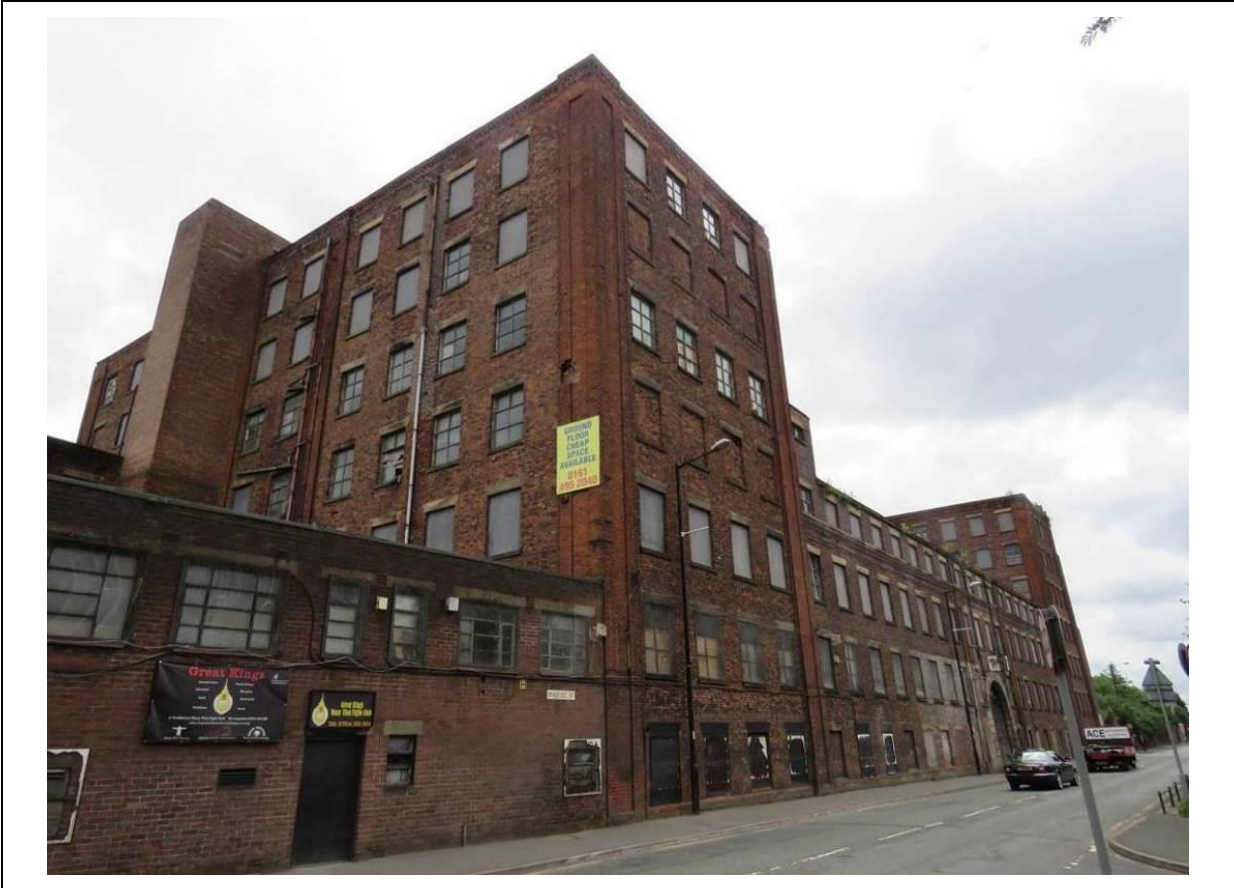
Figure 31 – Looking west along Bradford Road, showing the 1950s extension to the left.
